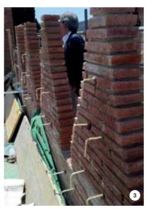
the battlements. The mesh - fastened to the vertical surfaces with MAPENET EM CONNECTOR - was applied in combination with MAPE-ANTIQUE HI-FLOW to strengthen the structure. The solution proposed by Mapei Technical Services. to apply a complete consolidation system comprising "reinforced" structural render on the mechanically weak masonry, managed to completely fulfil the expectations of the design engineers.
