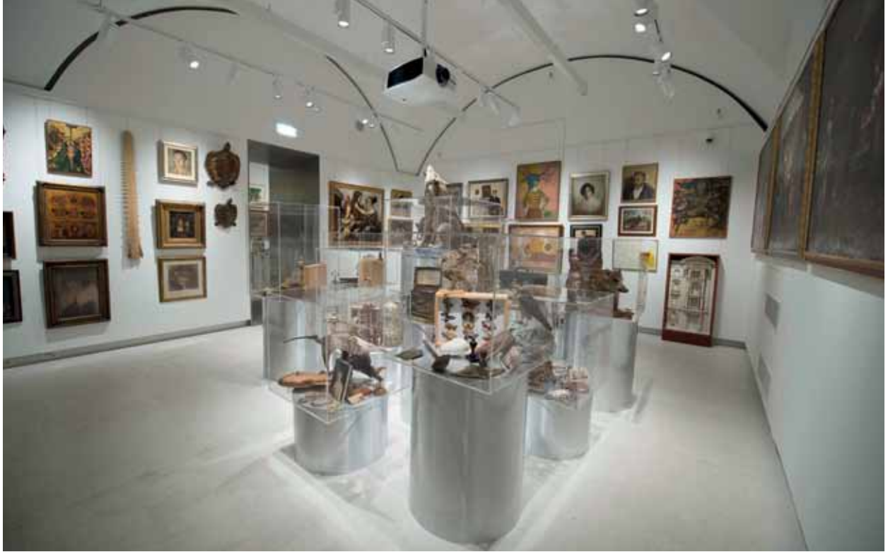
FIGURE 5. Applying the final protective paint SILEXCOLOR. FIGURE 6. Grinding of ULTRATOP 3 days after installation. FIGURE 7. Final polishing of the ULTRATOP SYSTEM "terrazzo alla veneziana" effect. IN THIS PAGE. The Rector's Palace has been officially opened in February this year.
