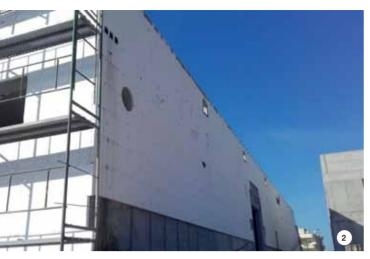
PHOTO 1. The Cretamel production unit in Heraklion, Crete. PHOTO 2. The external walls were properly insulated with the MAPETHERM EPS system before being finished with QUARZOLITE TONACHINO.
