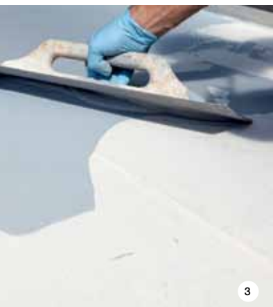
PHOTO 1. The first step was to prime the surfaces with MAPECOAT I 600 W.
