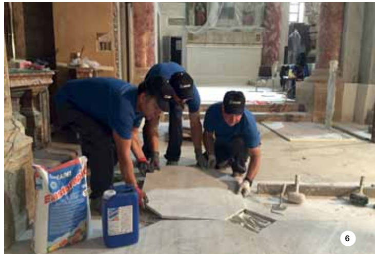
PHOTO 5. Static structural strengthening work on the dome over the presbytery using the MAPEWRAP system. PHOTO 6. The flooring, made up of slabs of Carrara marble and Bardiglio inserts, was installed using ELASTORAPID two-component cementitious adhesive.
