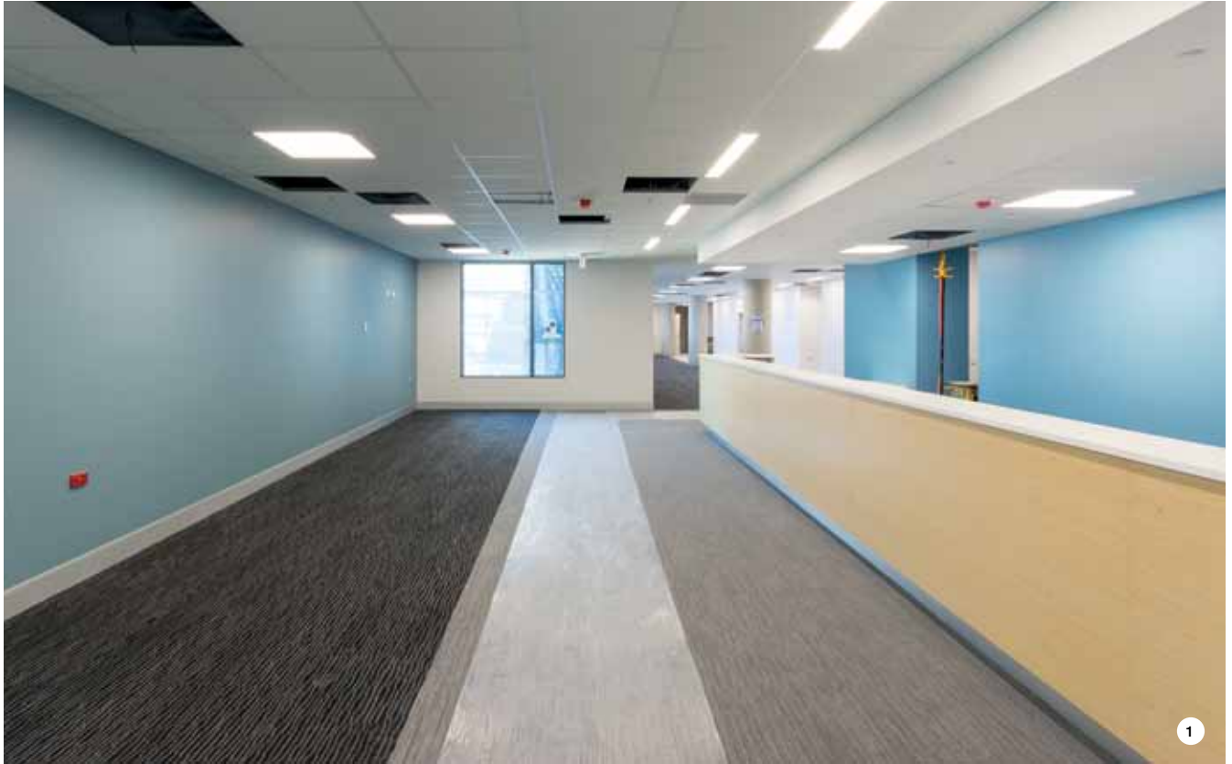
PHOTO 1. Substrates were treated with ECO PRIM T and levelled with ULTRAPLAN ECO before bonding the vinyl coverings with ULTRABOND VS90 PLUS.
