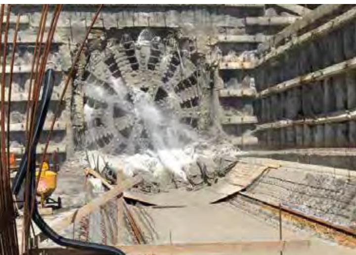
LEFT. The TBM breakthrough for the Santa Lucia tunnel took place on 8 th June 2022.
