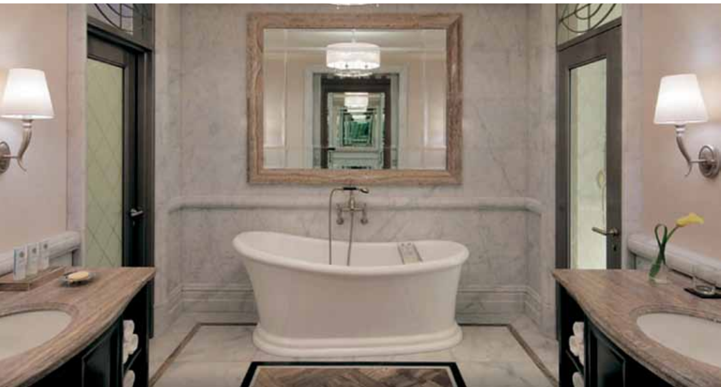
ABOVE. Ceramic tiles were installed with KERAFLEX MAXI S1, KERAFLEX and ADESILEX P9. BELOW. Substrates in the bathrooms were waterproofed with MAPELASTIC SMART and MAPELASTIC SEL.
