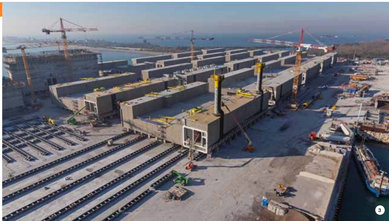
3. The precast concrete caissons being manufactured in the Malamocco site.
