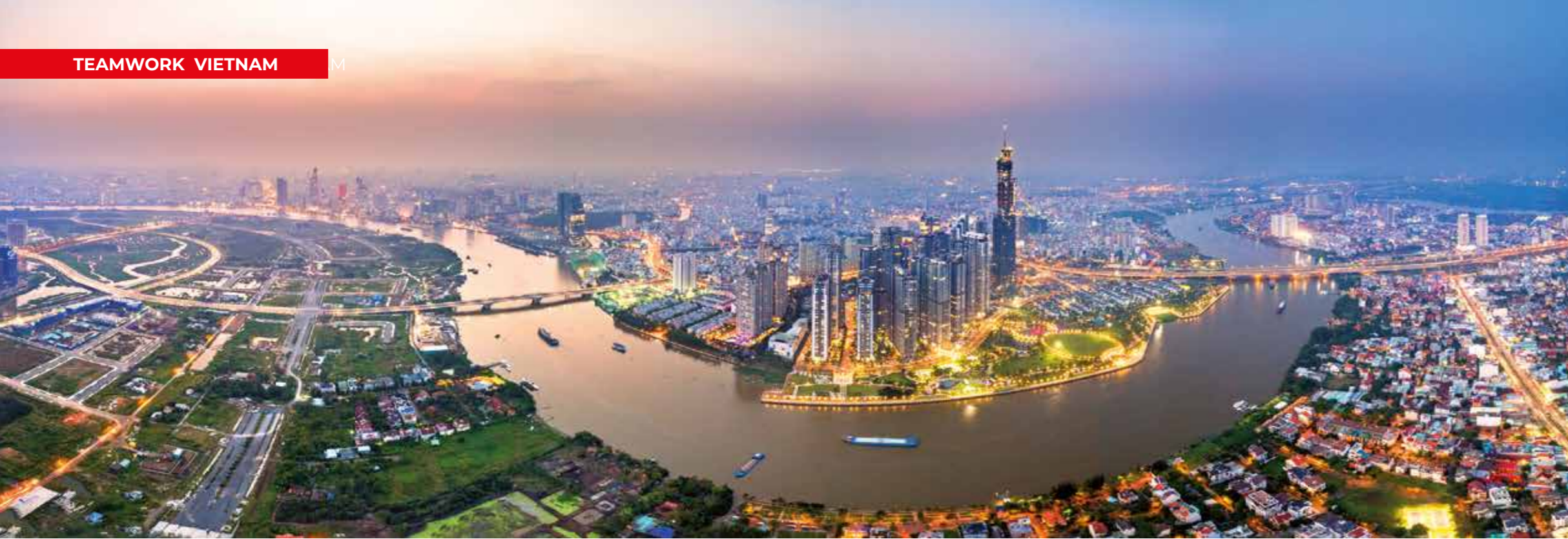
LEFT. The building industry has been growing fast in Vietnam for at least 10 years and is expected to continue to do so in the near future. ON THE OPPOSITE PAGE. The Mapei Vietnam manufacturing plant in Chu Lai, not far from Da Nang in central Vietnam, has been in operation since 2007.
