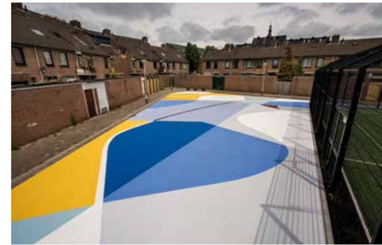
MAPECOAT TNS RACE TRACK was used to paint the asphalt surface. The synthetic grass for the playing area was installed using ULTRABOND TURF 2 STARS PRO two-component polyurethane adhesive.
