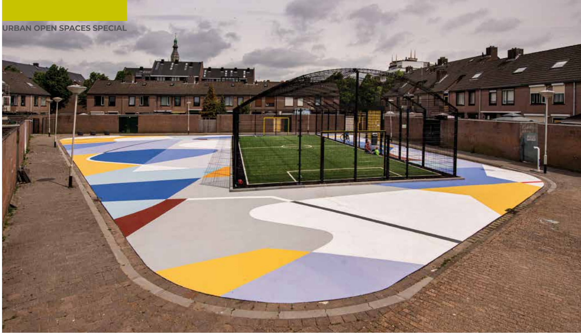
MAPECOAT TNS RACE TRACK was used to paint the asphalt surface. The synthetic grass for the playing area was installed using ULTRABOND TURF 2 STARS PRO two-component polyurethane adhesive.
