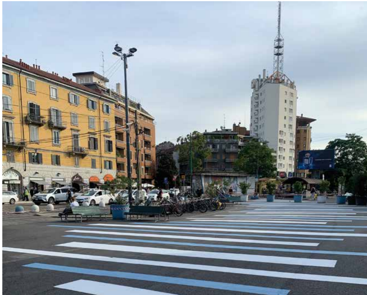
Two coats of MAPECOAT TNS EXTREME coloured epoxy-acrylic resin-based coating was applied on the surfaces of Piazzale Porta Genova. Work was completed by applying MAPECOAT TNS PROTECTION protective finish.
