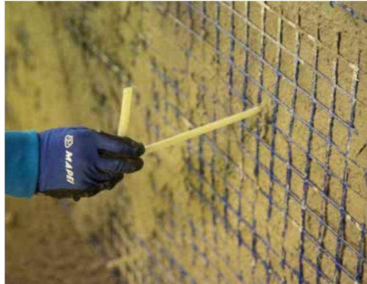
Detail view of the insertion of the MAPENET EM CONNECTOR within the CRM system.
