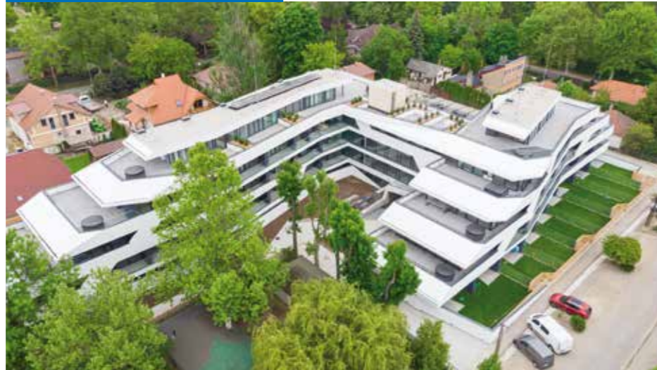
RIGHT. Mapei products were used for thermal insulation, finishing the façades, waterproofing the substrates and installing ceramic tiles in this residential complex shaped like a yacht in the town of Balatonszemes.
