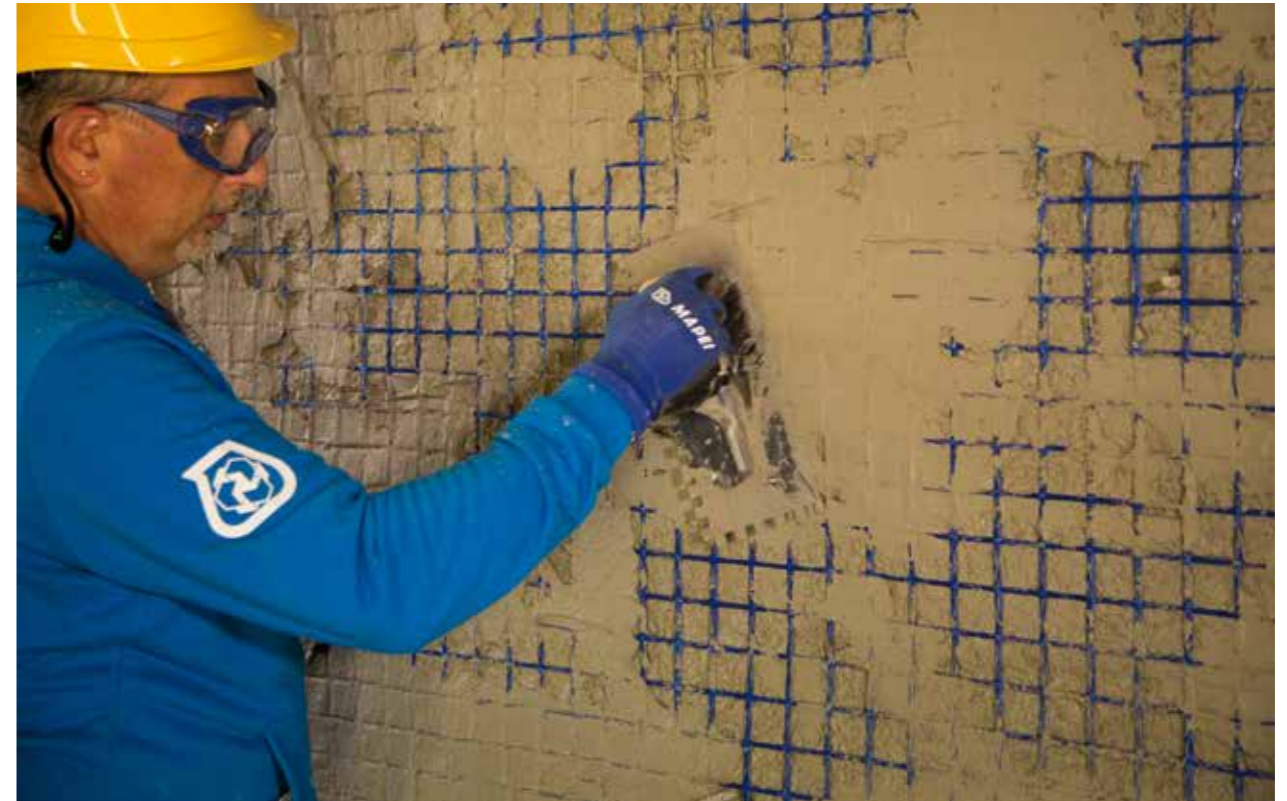
LEFT. Strengthening the extrados side of the vaulted ceiling of Palazzo Zicari Hotel in Matera (Italy). ABOVE. The meshes used in CRM strengthening systems increase overall strength and resistance and confine the elements to be reinforced.
