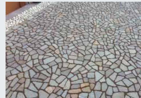
Paving made from assorted sizes of recovered cobblestones, cubes and irregular stone units sealed with MAPESTONE JOINT.
