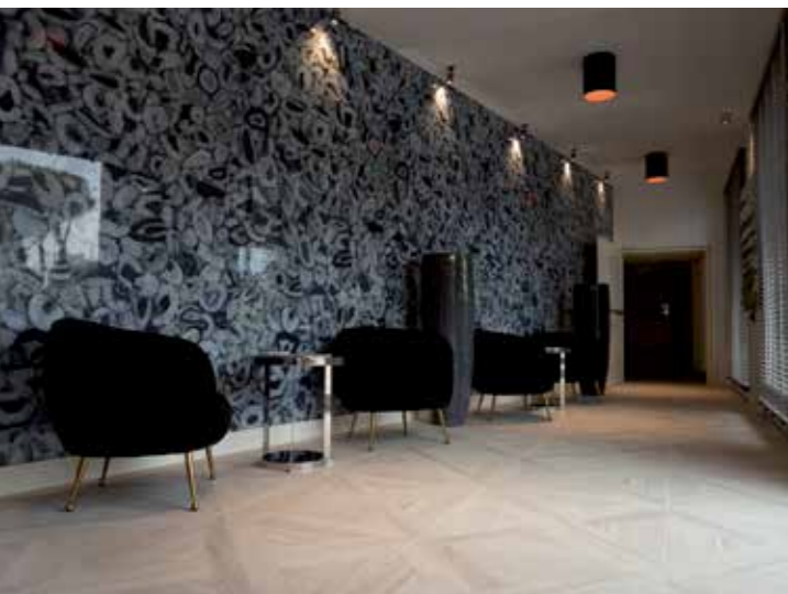
LEFT. In the corridor that connects the two structures, large Fiandre tiles (measuring 150 x 320 cm) were installed on the walls with ULTRALITE S1 adhesive. RIGHT. In the wellness area, large-size ceramic tiles were bonded on the floors with KERAFLEX EASY S1 adhesive.
