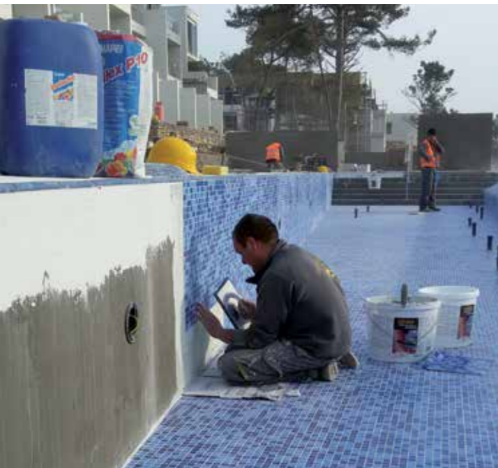
ABOVE. Wood-effect porcelain tiles were bonded with KERABOND PLUS in the old pavilion rooms, while mosaic tiles were installed in the outdoor pool with ADESILEX P10.
