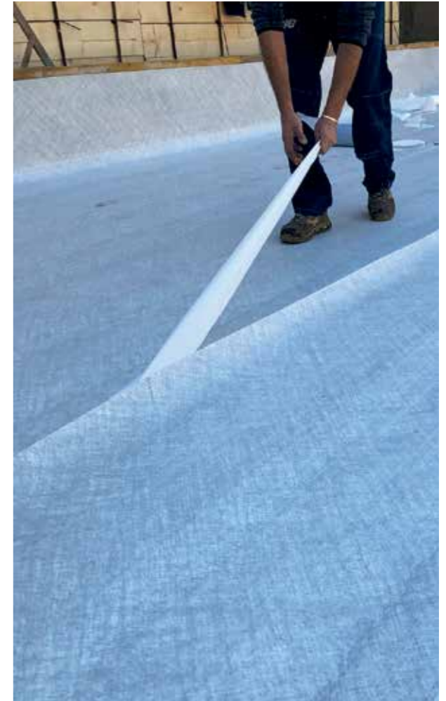
Waterproofing horizontal surfaces with Mapei fully-bonded membranes.
