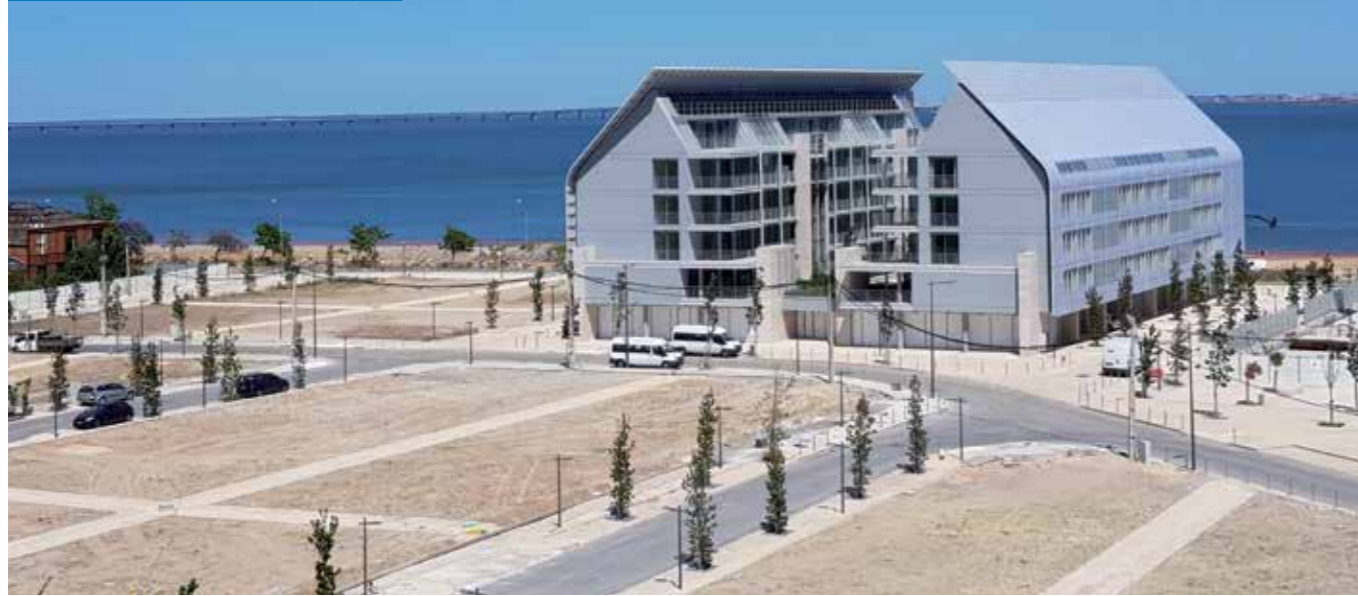
ABOVE. The Prata Living Concept residential complex in Lisbon, designed by Renzo Piano and completed with Mapei solutions.
