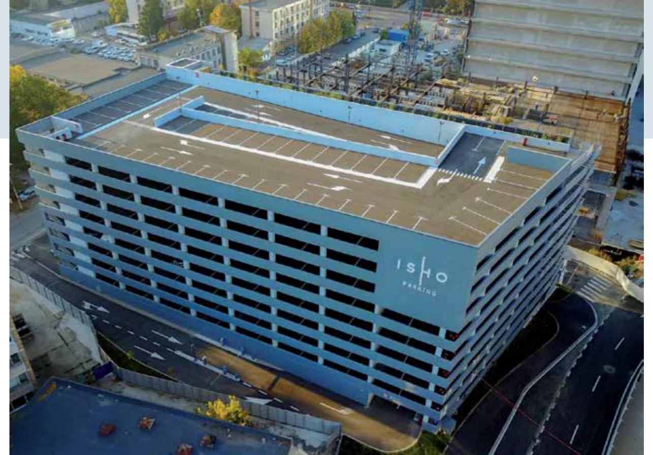
A view of the multi-storey carpark in the Isho neighbourhood in Timisoara whose roofs were waterproofed with POLYBOND HP P.
