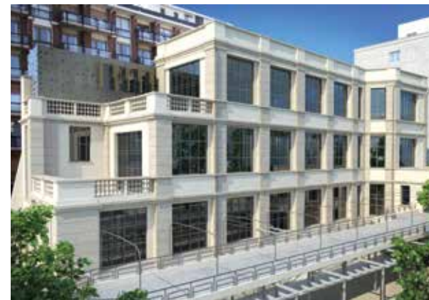
For the restoration of the Artists' House, one of the first buildings (1909) constructed in Milan using the brick and concrete method, it was decided to conserve the original structure and to insert an internal steel exoskeleton to give it the static and anti-seismic properties required by current standards. Mapei supplied products for the refurbishment, conservative restoration and protection of the masonry.
