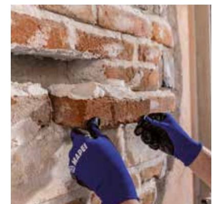
Rebuilding brick masonry
