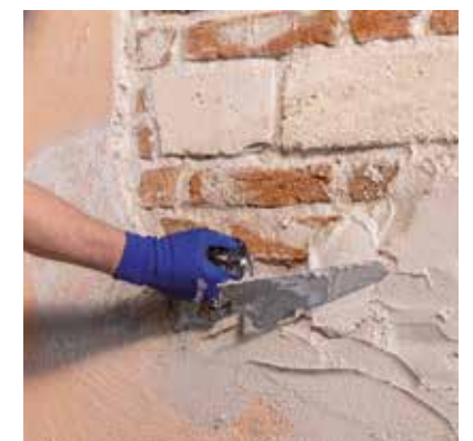
Levelling off and repairing render
