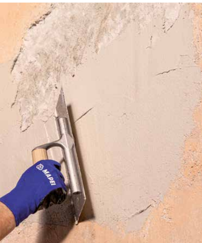
MAPE-ANTIQUE NHL ECO RESTAURA is a multi-purpose, cement-free mortar made from natural hydraulic lime and Eco-Pozzolan.
