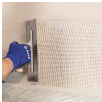
Positioning an alkali-resistant glass fibre mesh on the first skim coat.
