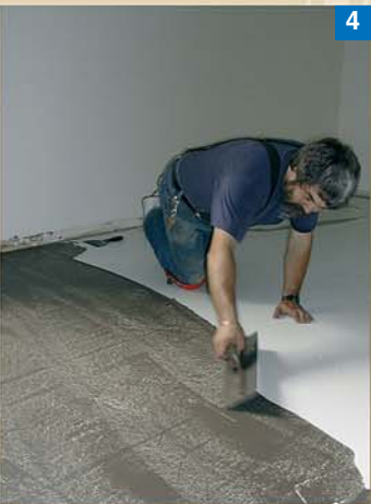
Photo 4. Planipatch Plus System was applied on the substrates, which had been previously treated with Planiseal MRB.
