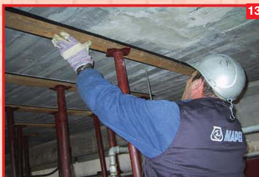
Photo 13. Reinforcing the floor slab.
