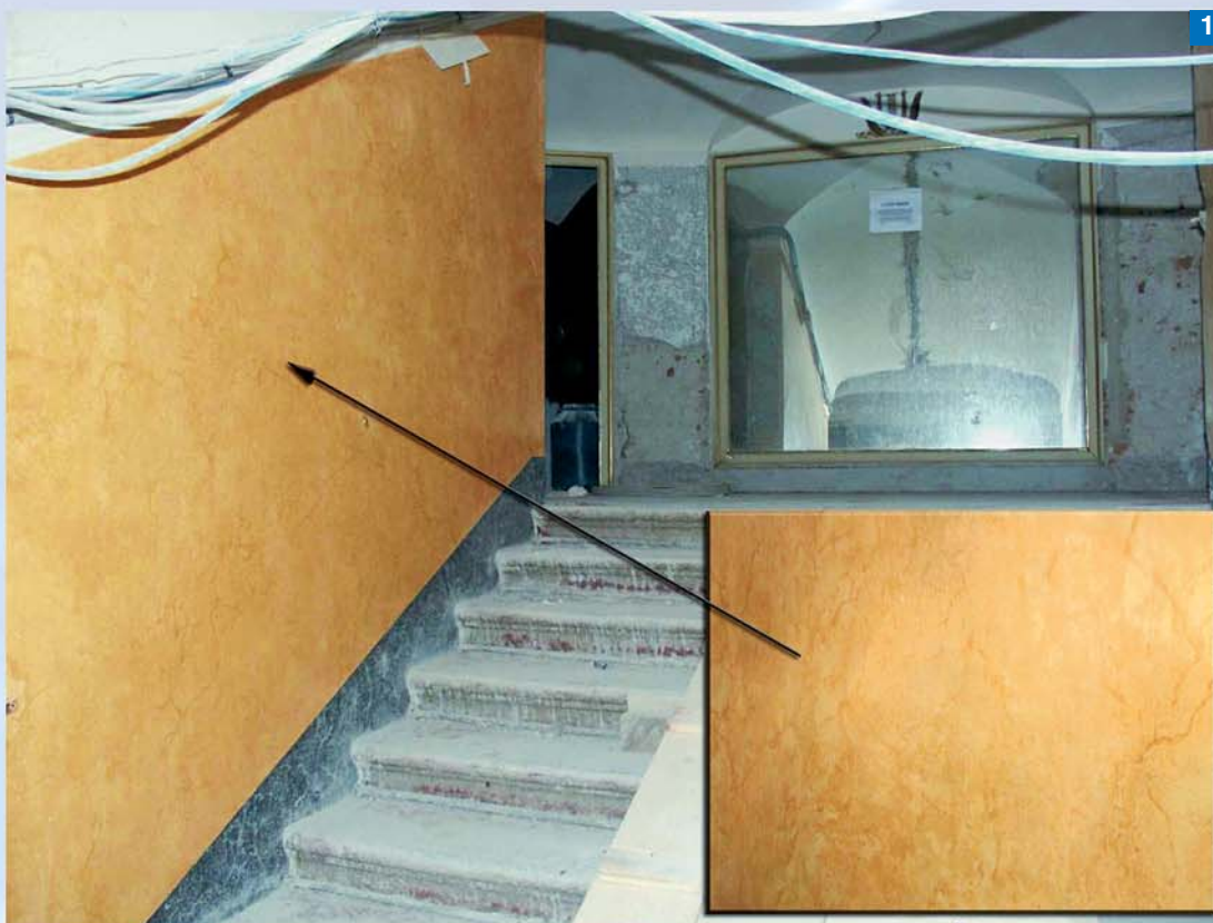
Photo 1. Interior of the Teatro alla Scala in Milan: the insert in the bottom right corner shows a detail of the Piermarini marmorino, the original wall coating, which has been covered with several coats of paint.
