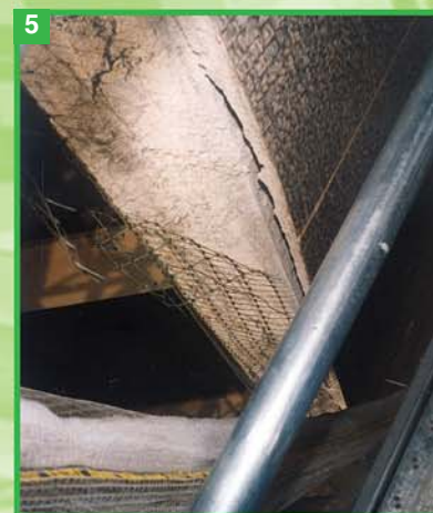
Photo 5. Partial detachment of the installation mortar from the underlying levelling concrete without the collapse of the glass mosaic.
