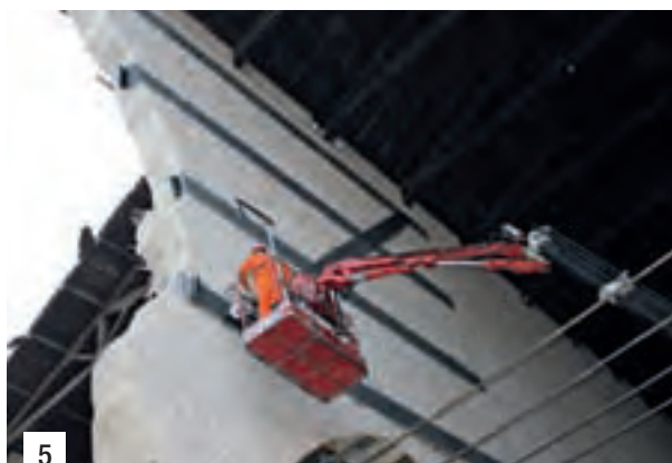
Photo 3. Spreading on a layer of MAPEWRAP 31 epoxy adhesive.
