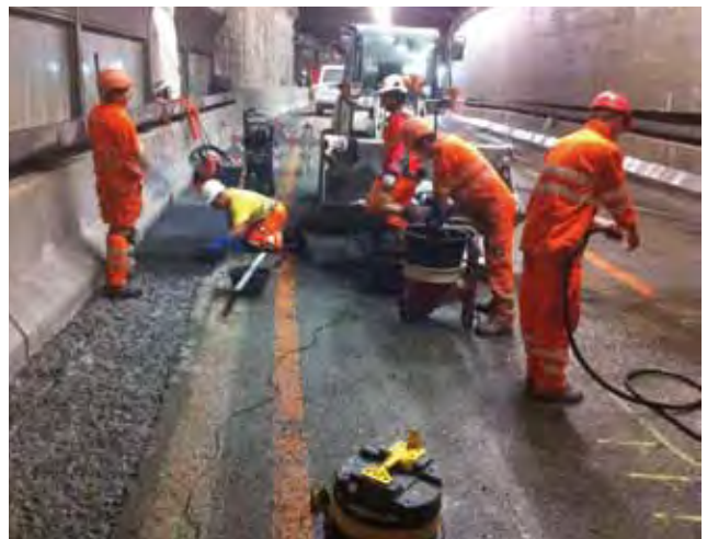
BELOW LEFT. Anchoring metal elements with PLANITOP FIX. BELOW RIGHT. Reconstruction of the surface patches on the carriageway of the bridge connecting the two tunnels with MAPEGROUT SV and MAPEGROUT SV T.
