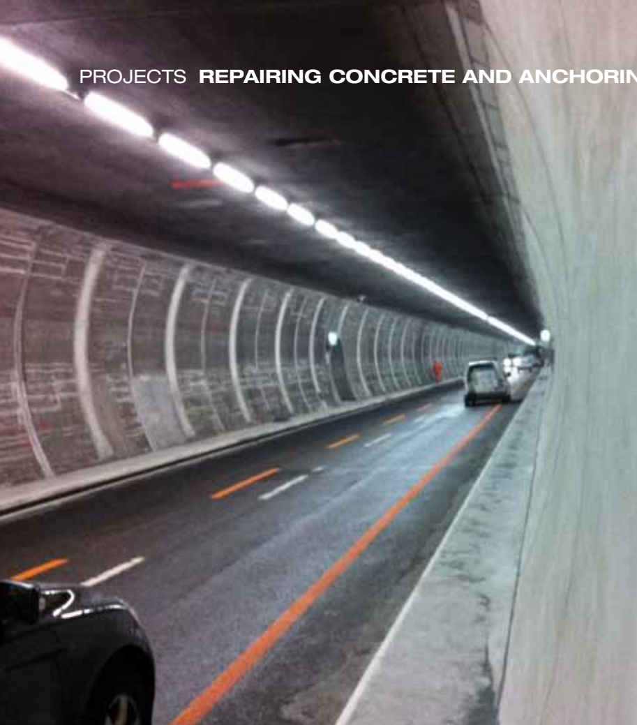
ABOVE. The walls inside the tunnels after applying MAPEFINISH two-component mortar.
