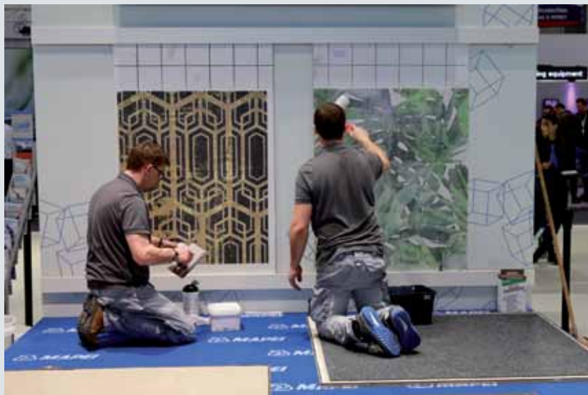
At Domotex 2020 Mapei technicians showed the application of the Decor line products for wallpaper.
