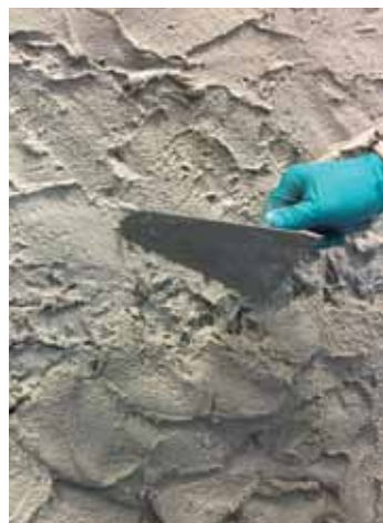
Applying POROMAP DEUMIDIFICANTE by trowel.
