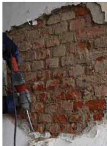
Removing the deteriorated render.
