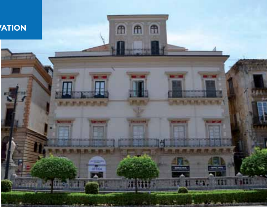
ABOVE. The palace after completion of the works. LEFT. After removing the detached masonry and renders and cleaning the substrates, the façades were painted and protected with SILANCOLOR BASE COAT and SILANCOLOR PAINT PLUS.
