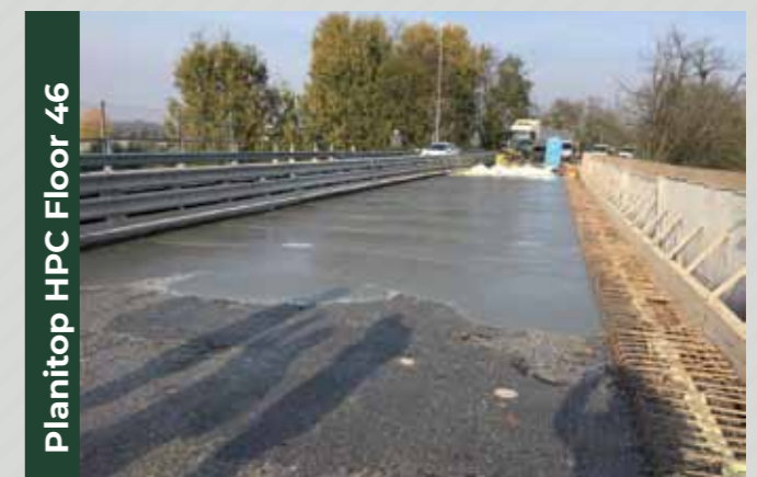
Repairing a road surface with PLANITOP HPC FLOOR 46.
