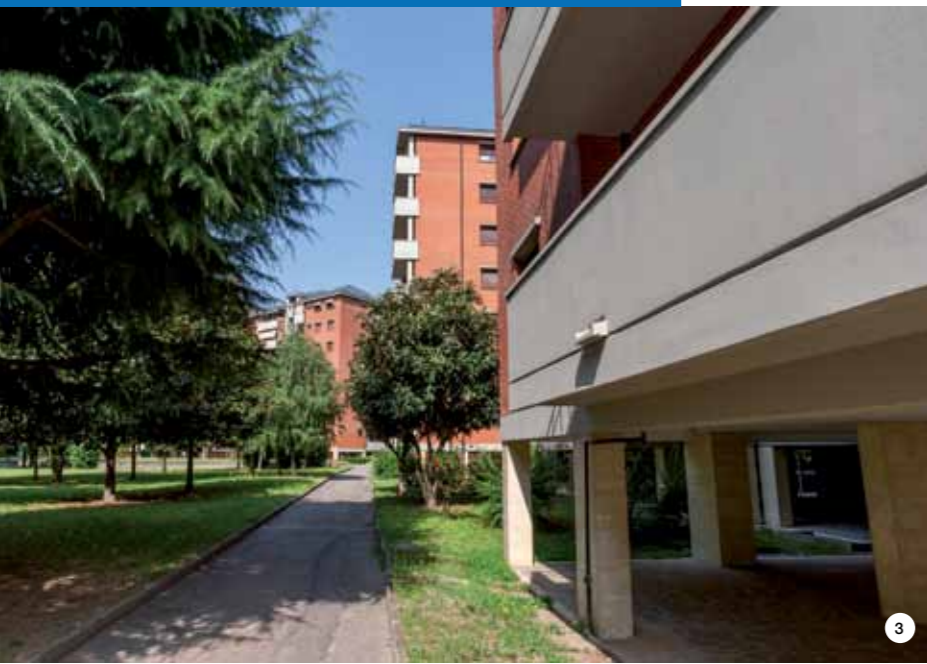
3. The MAPETHERM external thermal insulation system was recommended for the pilotis floor.
