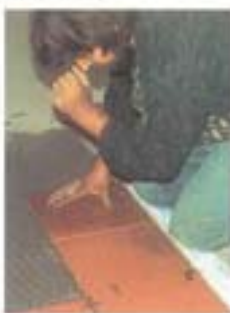
PHOTO 3 Setting terra cotta tiles
