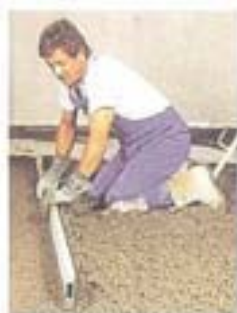
PHOTO 1 Screeding with MAPECEM
