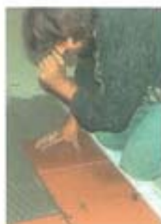
Setting terra cotta tiles
