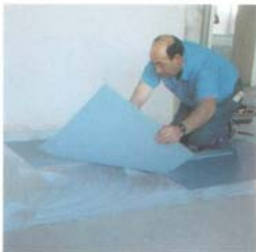
Setting PVC floors on a MAPECEM screed and, below, the look of the room once done
