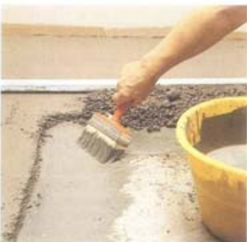
Pouring the slurry bond coat for anchoring adhering Mapecem screeds
