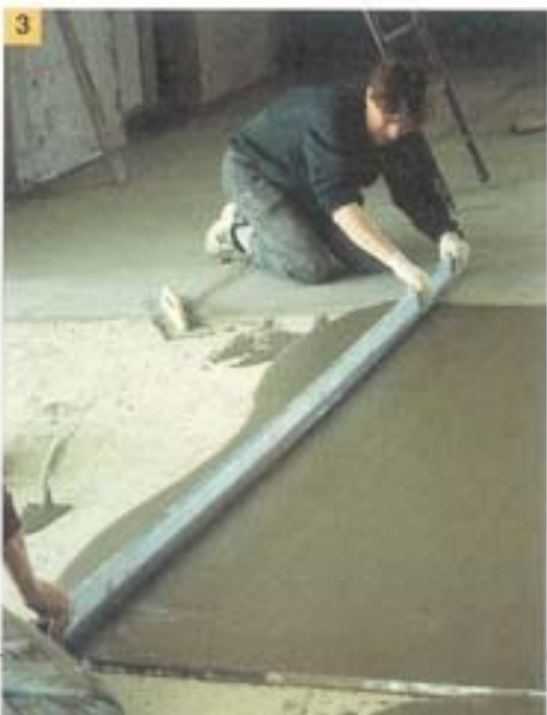
Photo 3: straight-edging of the ADESILEX P4* levelling compound.
