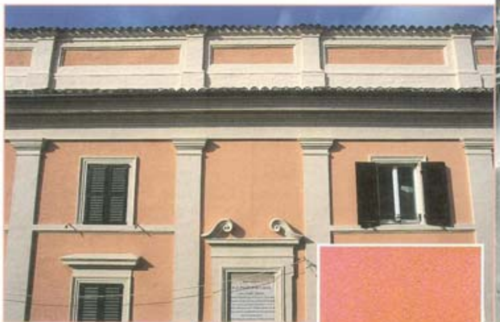
Collegio Gentile, Fabriano (Ancona - Italy). The close-up shows the grain of the SILEXCOLOR TONACHINO used for the finish.
