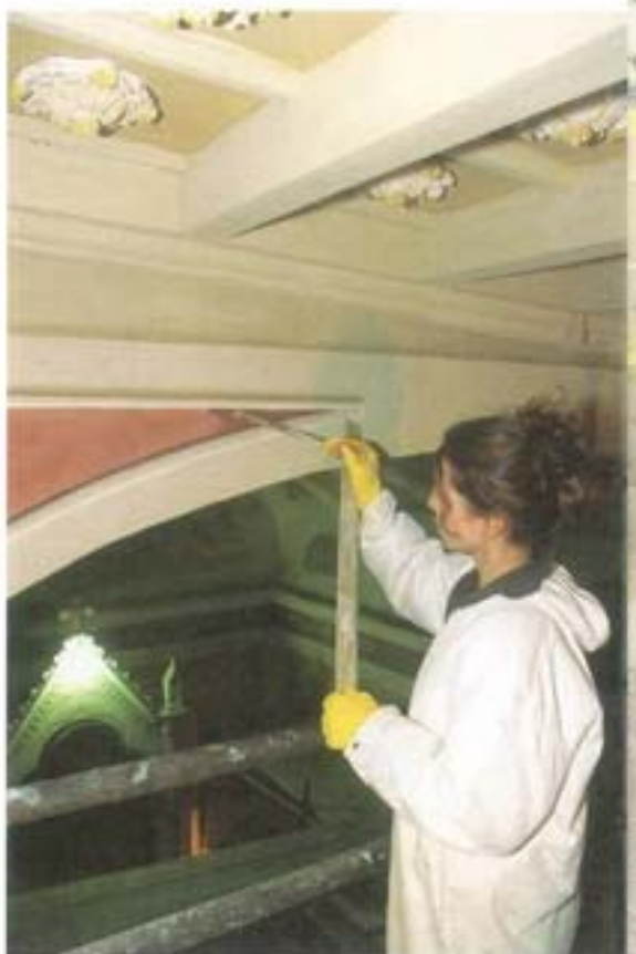
Church in Merone (Como - Italy). Detail of a finish applied to the interior using SILEXCOLOR TONACHINO.
