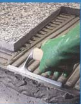
Installation of tiles with external middlings.
