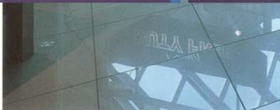
Figure n. 1 - Installation of 40x40 marmorized porcelain tile on an internal wall. Adhesive: KERAFLEX MAXI. Grout: ULTRACOLOR.
