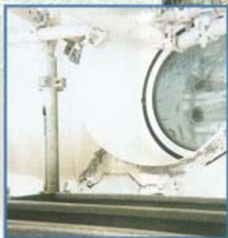
Photo 2. Processing one of the new openings carried out on the building shaft.
