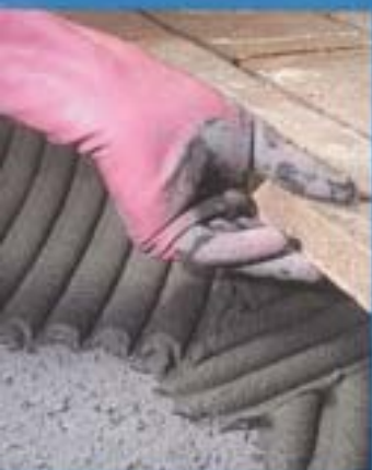
Baked tile installation done by hand on an irregular screed.
