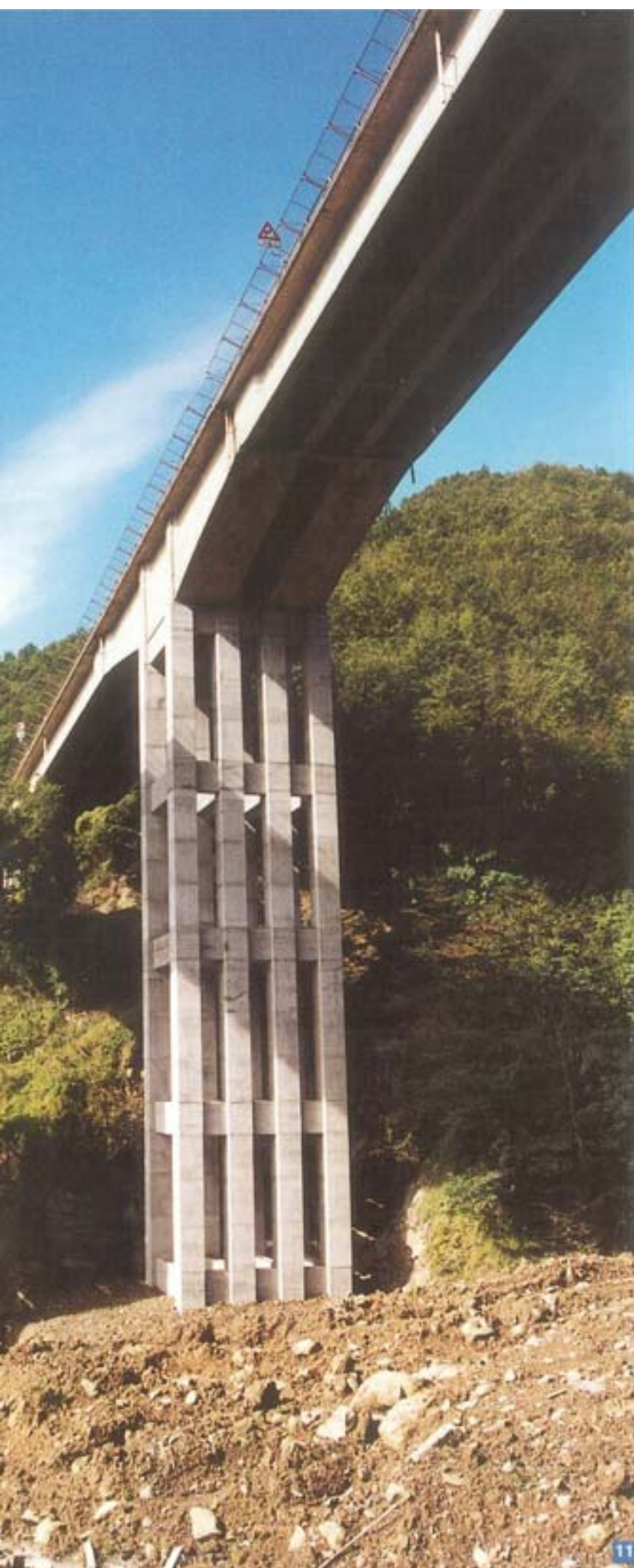
Photo 11. The viaduct at the completion of the recovery intervention.
