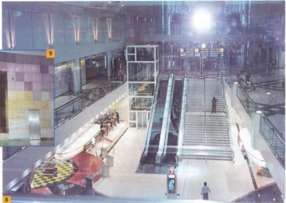
Photo 8. The connecting stairs were covered with granite using KERALASTIC.
