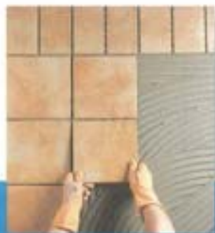
Installation of klinker tiles outdoors.
