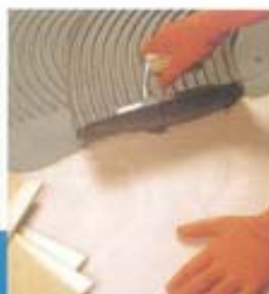
Laying porcelain tiles on multi-layered marine plywood substrate.
