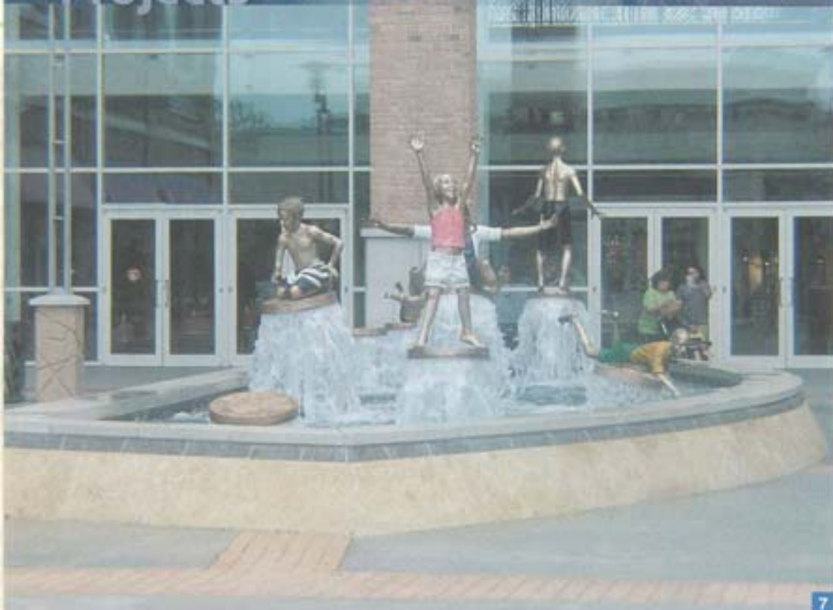
Photo 7. The heart of the "village", made of a covered structure, is behind the decorative fountain.
