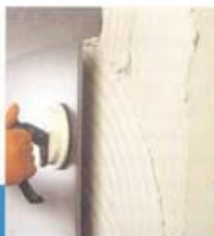
Laying large porcelain tiles over a concrete façade.
