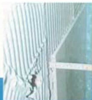
Thickly applied porcelain wall tiles.
