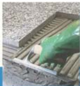
Installation of marble-chip "graniglie" tiles outdoors.
