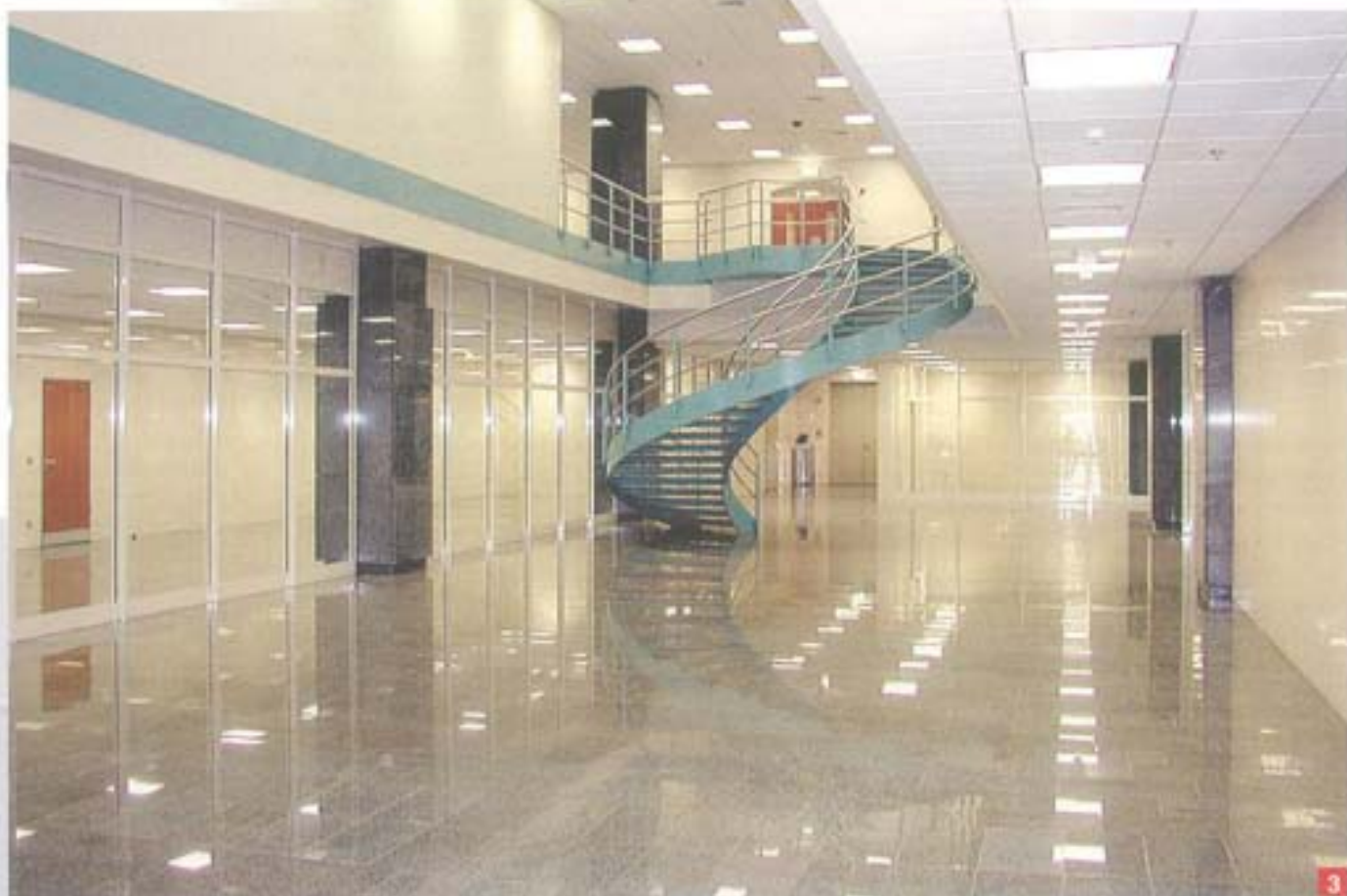
Photo 5. Azul Montana granite was chosen for the counters area and installed using Keraquick.
