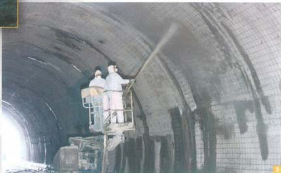
Photo 3. Technicians busy spraying on Mapegrout Gunitite. You can clearly see the electrically welded steel mesh forming the frame for the plaster made from Mapegrout Gunitite. The product was applied using a rotary pump directly supplied by bags of dry product hydrated when emerging from the hose.
