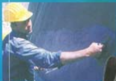
Application by trowel
