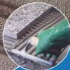
Laying marble-chip embossed terrazzo tiles for outdoor use
