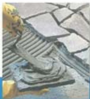
Installation of hewn back stones with buttering.
