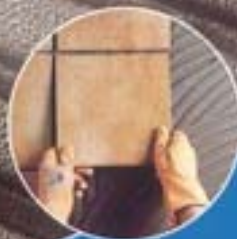
Laying klinker tiles for outdoor use
