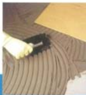
Spreading Elastorapid over a cement-based screed with a notched trowel.
