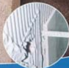
Thick laying porcelain tiles on walls
