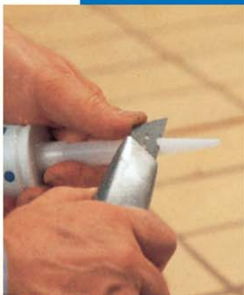
Cutting the nozzle according to the size of the joints.
