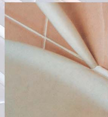
Sealing sanitary ware.
