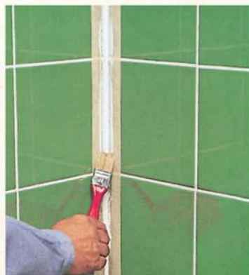
Smoothing the joint with soapy water and a small brush.
