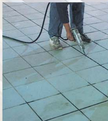
Sealing a ceramic tile floor with Mapesil AC.
