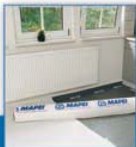
Fixing Mapetex on Mapetex-Strip
