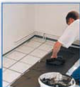
Installing ceramic tiles with Keraquick
