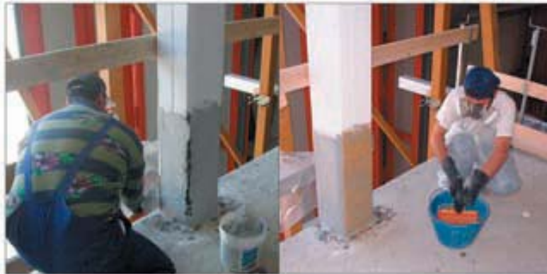
Application of grout
