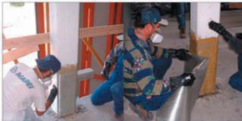
Application of the first layer
