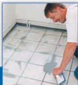
Grouting with Ultracolor Plus
