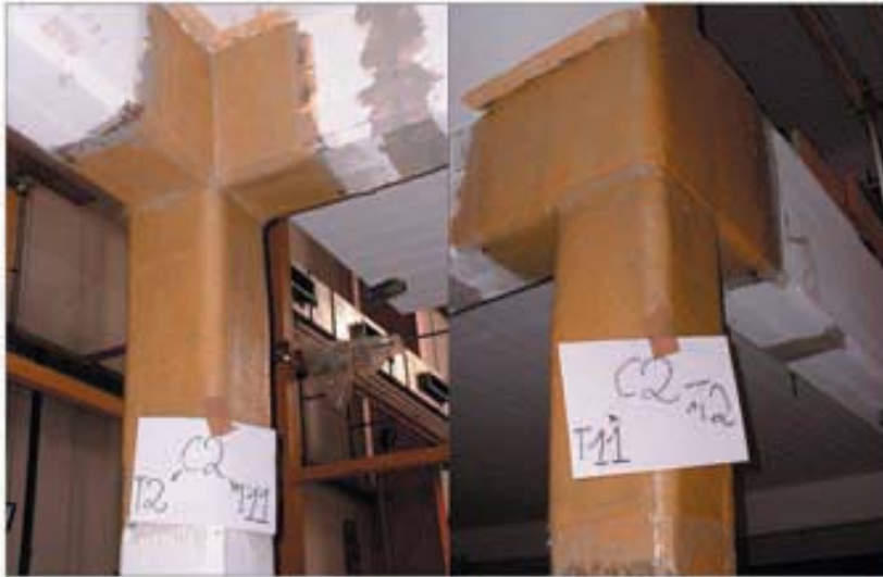
Internal view of the joint
