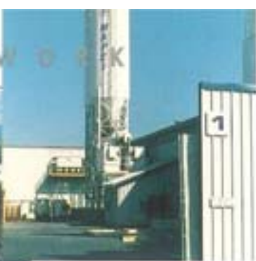
On the left the plant of Vancouver and here below a few images of the plant and of the laboratory in Laval
