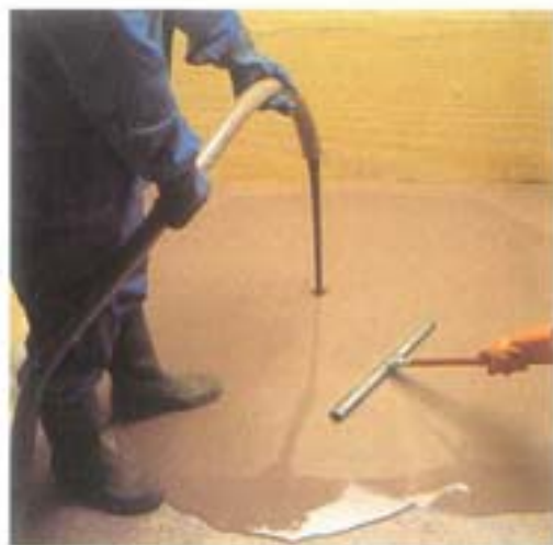
Leveling with ULTRAPLAN. A pump was used for the application.
