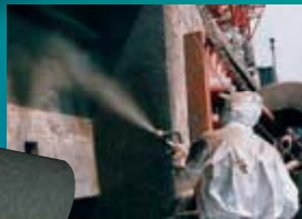
Application by spraying
