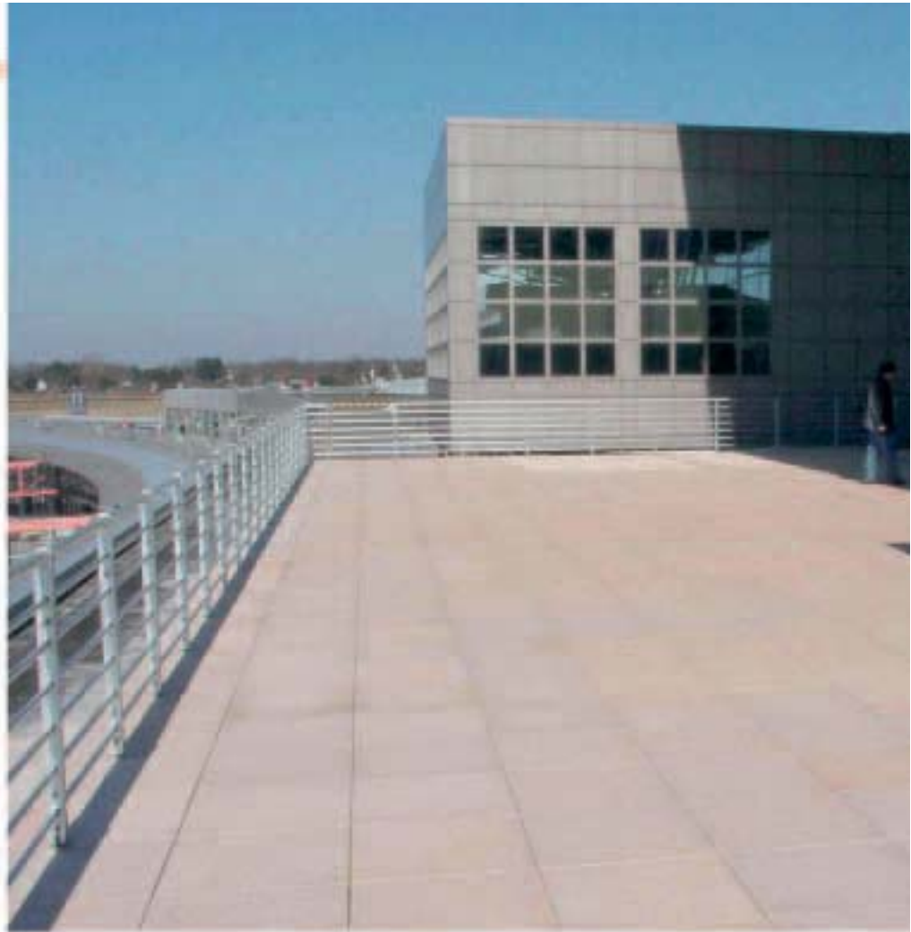
Photo 3. Padang yellow granite slabs were laid on the terrace's floor with a drainage mortar formulated with the hydraulic binder Mapecem. On the back of the slabs, Granirapid two-component cementitious adhesive was also applied.
