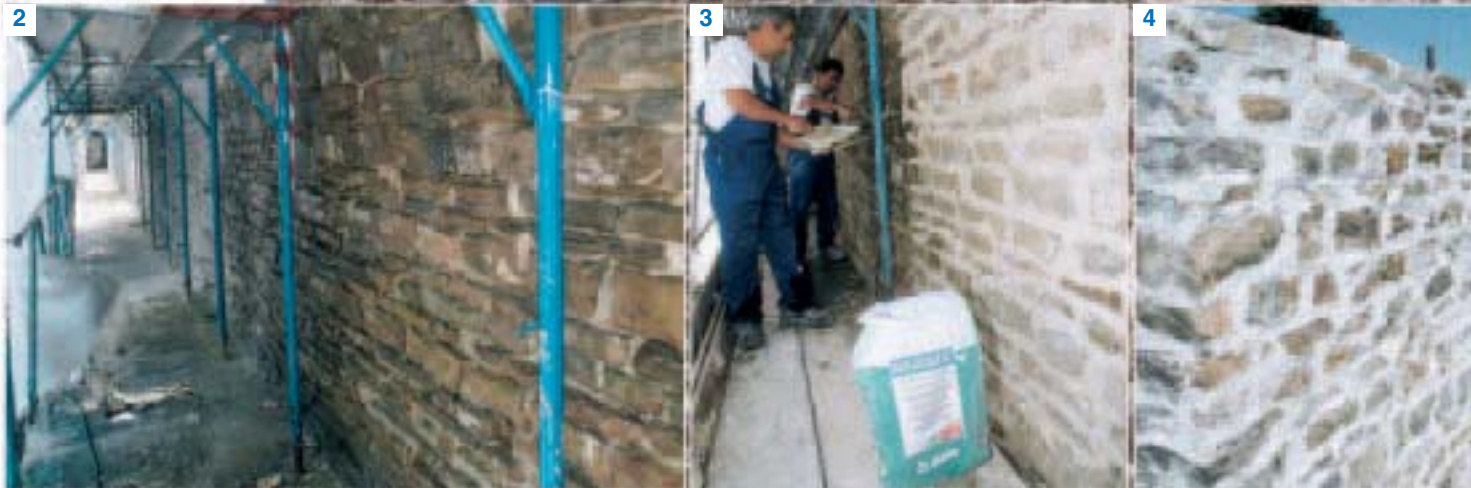
Photo 4. Detail of the walls after completing the work.
