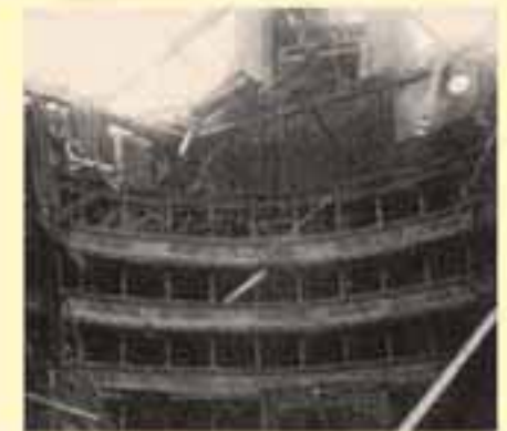
The Teatro alla Scala in Milan with serious damages due to the Second World War bombing.
