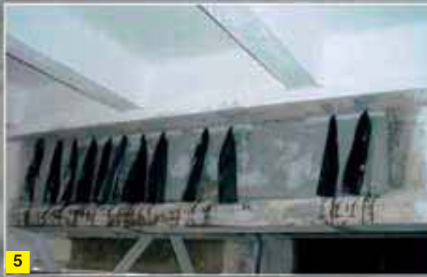
Photo 5. Positioning anchoring ties made from portions of MapeWrap C UNI-AX 300/20.
