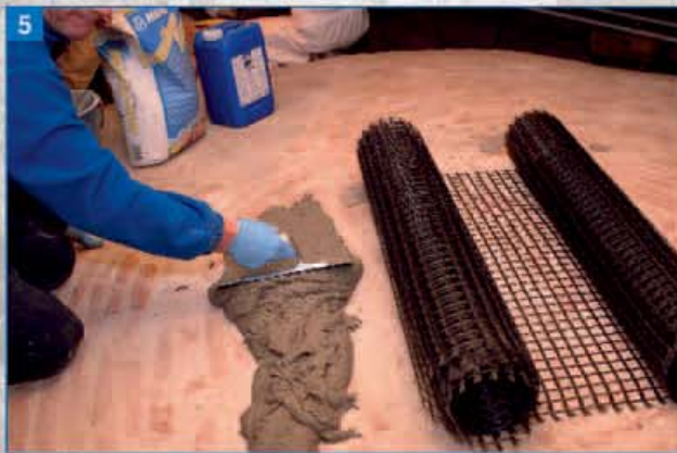
Photo 8. Application of the second layer of Planitop HDM.
