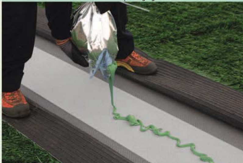
Application of Ultrabond Turf PU 1K on the jointing tape by extrusion from its aluminium packaging
