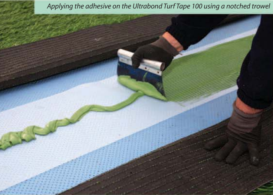
Bonding the jointing strips between the synthetic grass panels
