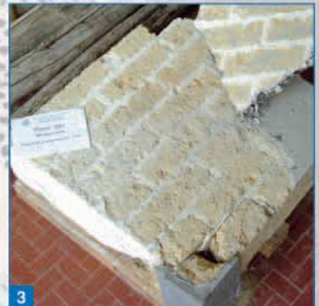
Photo 1. Failure mode of a panel without strengthening.
