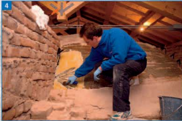
Photo 4. Application of MapeWrap C Fiocco.
