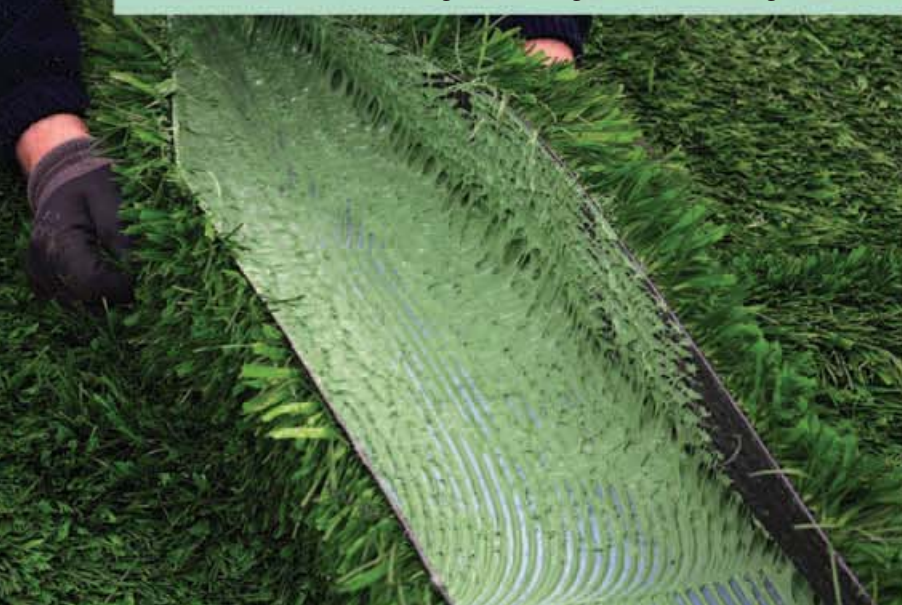
Checking the buttering on the back of the grass surface
