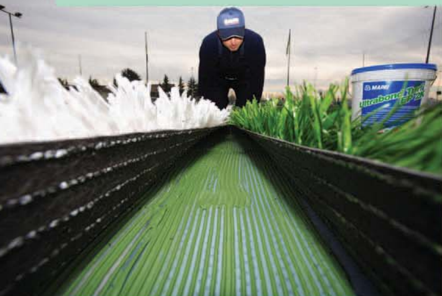
Checking the buttering on the back of the grass surface
