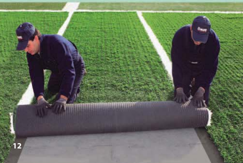
Synthetic grass rolls being acclimatised before laying
