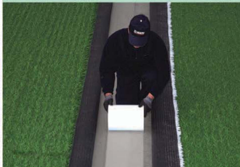
Laying the Ultrabond Turf Tape 100 jointing tape
