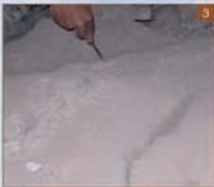
Photos 3 and 4. The cracks in the vaulted roof above the Ball Hall were opened and then sealed using Eporip adhesive.
