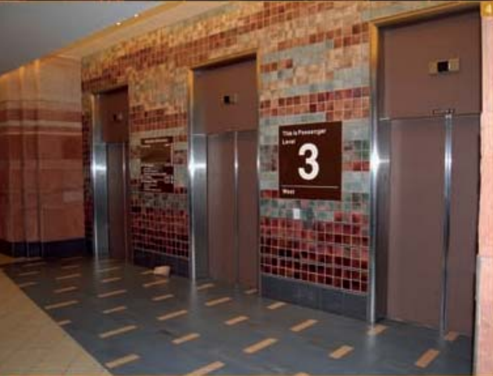
Photo 4. Glazed clay tiles were bonded on the elevators' external walls with Kerabond adhesive, mixed with Keralastic admixture (which is the American equivalent of Isolastic).
