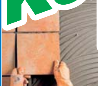
External installation of clinker tiles
