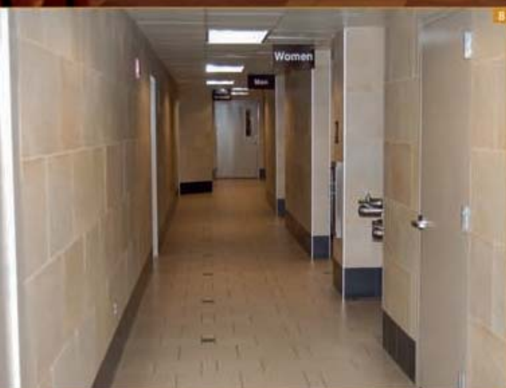
Photos 7 and 8. Porcelain tiles were laid on the toilettes' walls and floors with Kerabond+Keralastic, after waterproofing the substrates with Mapelastick 315 cementitious membrane.
