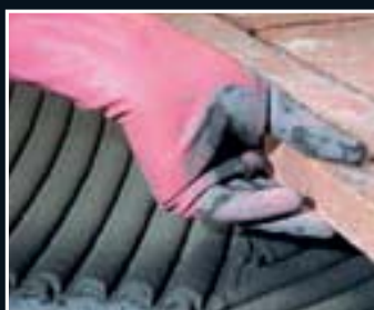
Installation of hand made terracotta tiles on an uneven screed
