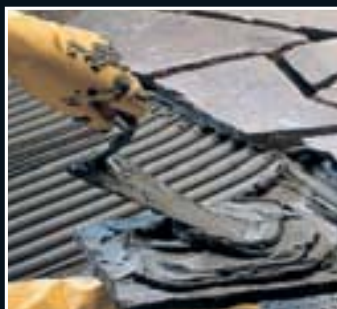
Installation of external hewn back stone with buttering
