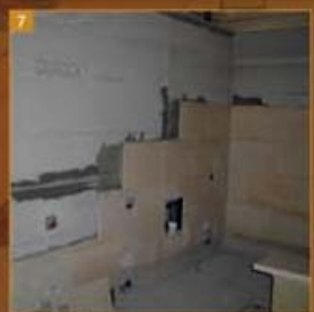
Photos 7 and 8. Porcelain tiles were laid on the toilettes' walls and floors with Kerabond+Keralastic, after waterproofing the substrates with Mapelastick 315 cementitious membrane.
