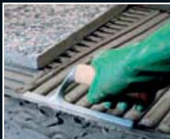
External installation of relief terrazzo "graniglie" tiles
