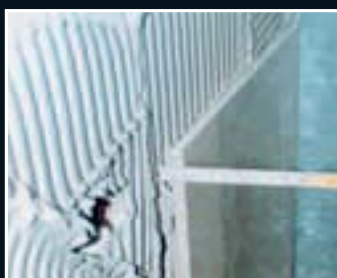
Thickly applied porcelain tiles on a wall
