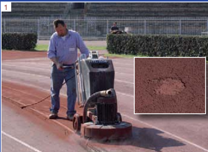
Photo 1. Mechanical grinding of the old surface with a close up of the deterioration of the old covering.
