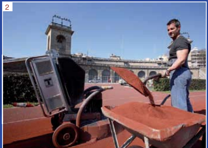
Photo 2. Reclaiming the ground-off material.
