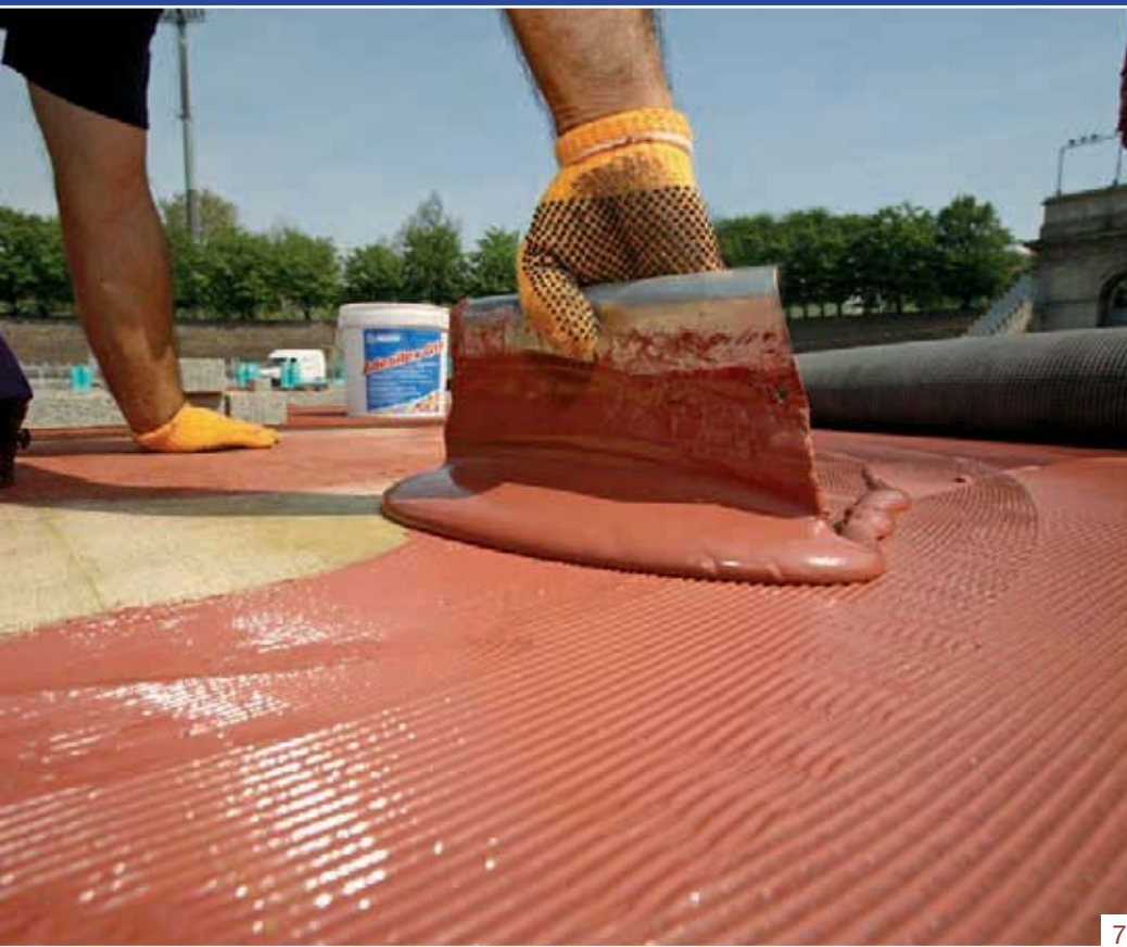
Photo 3. Mixing Adesilex G20 with ground rubber removed from the old track.
