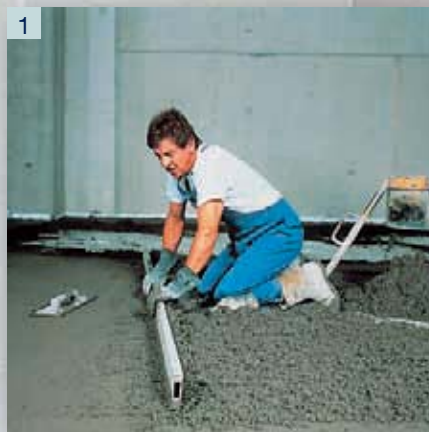
Photo 1. Preparation of a cementitious screed with Mapecem binder.
