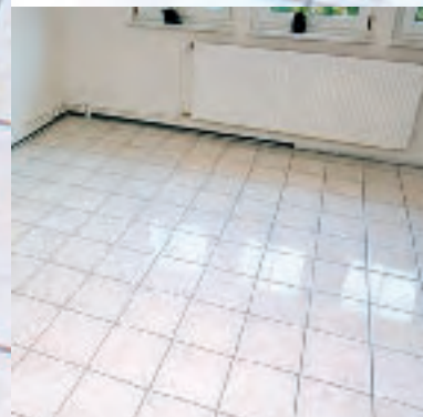
Removable flooring installed with Mapetex System
