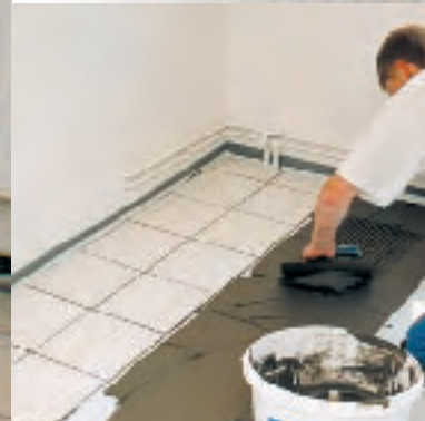
Installing ceramic tiles with Keraquick
