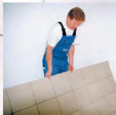
Removing a ceramic floor installed with Mapetex System
