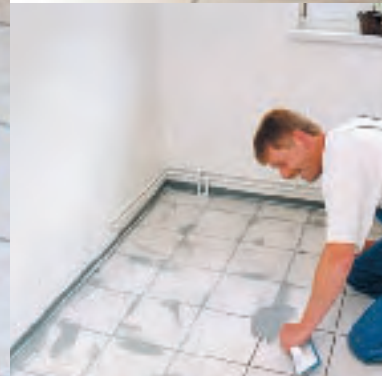
Grouting with Ultracolor Plus
