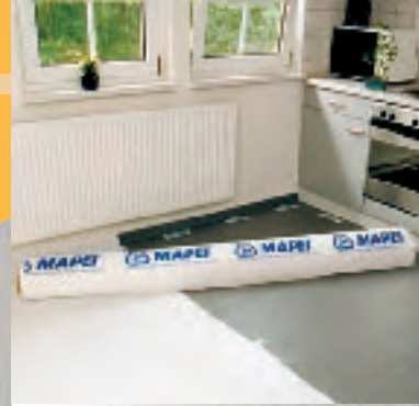
Fixing Mapetex on Mapetex-Strip
