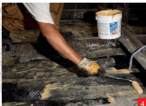
Photo 5. Preparation work before laying MapeWrap C UNI AX.
