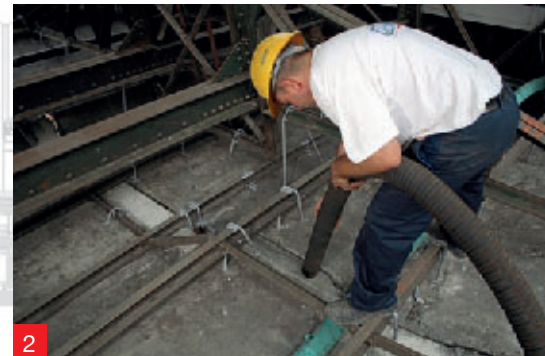
Photo 4. Applying MapeWrap 31 adhesive.
