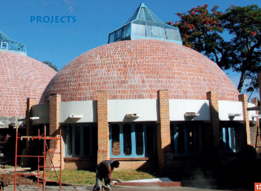
Photo 13. The parts of the structures covered with ceramic tiles were protected using Antipluviol S and Antipluviol W colourless impregnating solutions.
