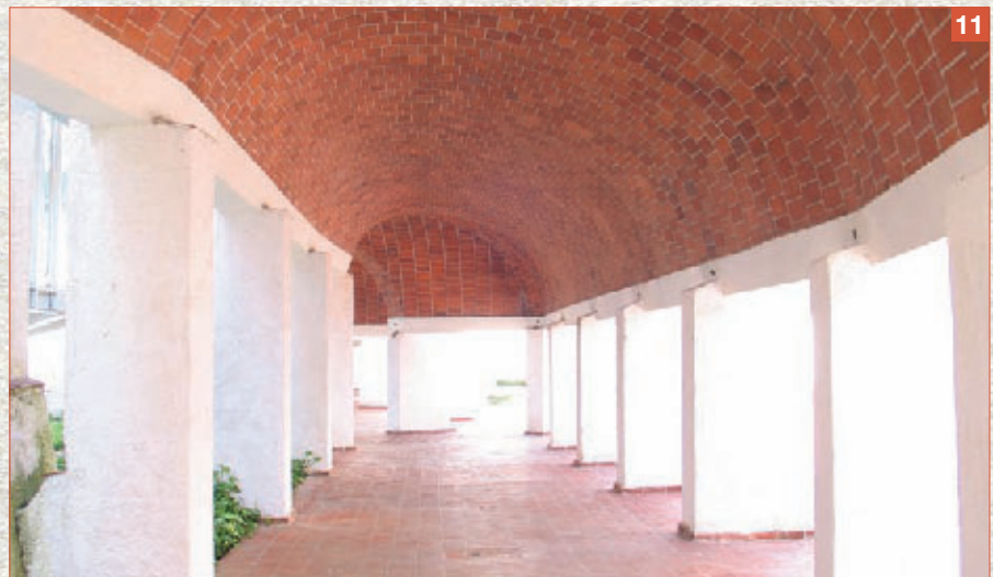
Photos 10 and 11. Inside the buildings, the pillars on which the vaulted roofs of the bòvedas and cupolas are positioned, were initially consolidated by injecting Mape-Antique I. The tiles were then laid using Kerabond+Isolastic. The tile joints were then grouted with Keracolor GG and Ultracolor.
