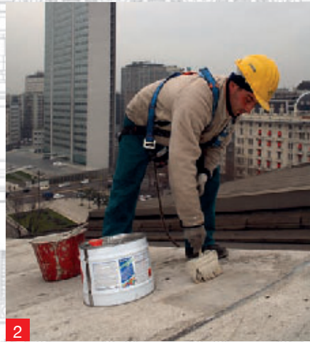
Photo 1. Monolithic sealing of the blocks with Mapesil BM.
