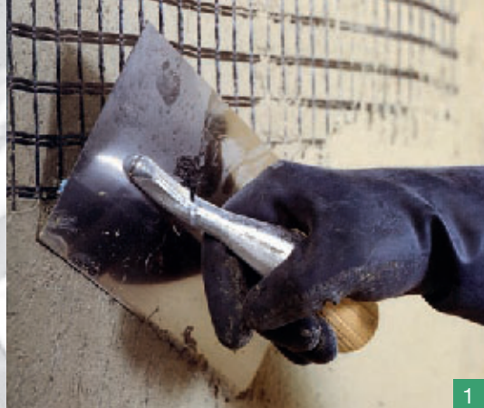
Photos 3 and 4. Binding pillars and beams with MapeWrap System.
