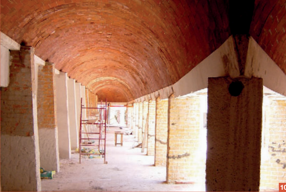
Photos 10 and 11. Inside the buildings, the pillars on which the vaulted roofs of the bòvedas and cupolas are positioned, were initially consolidated by injecting Mape-Antique I. The tiles were then laid using Kerabond+Isolastic. The tile joints were then grouted with Keracolor GG and Ultracolor.
