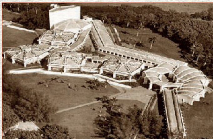
The School of Modern Dance Before Renovation
