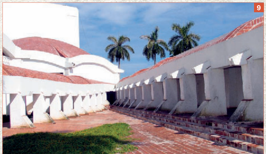
Photo 9. The restored surfaces were smoothed and levelled with Mapefinish mortar mixed with Planicrete latex.
