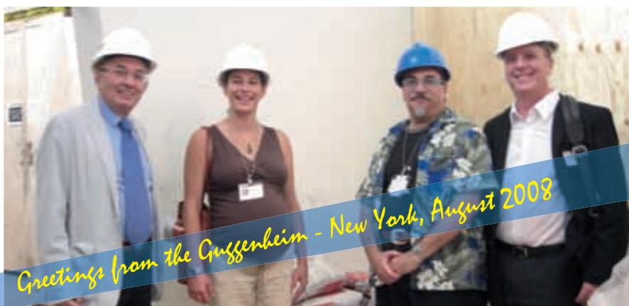
At the building site: from left, Giorgio Squinzi, Amanda Thomas-Trienens (ICR), Norman Weiss (Columbia University) and Bruce Burton (Mapei Corp.).
