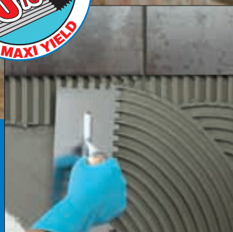
Application of Ultralite S1 with notched trowel
