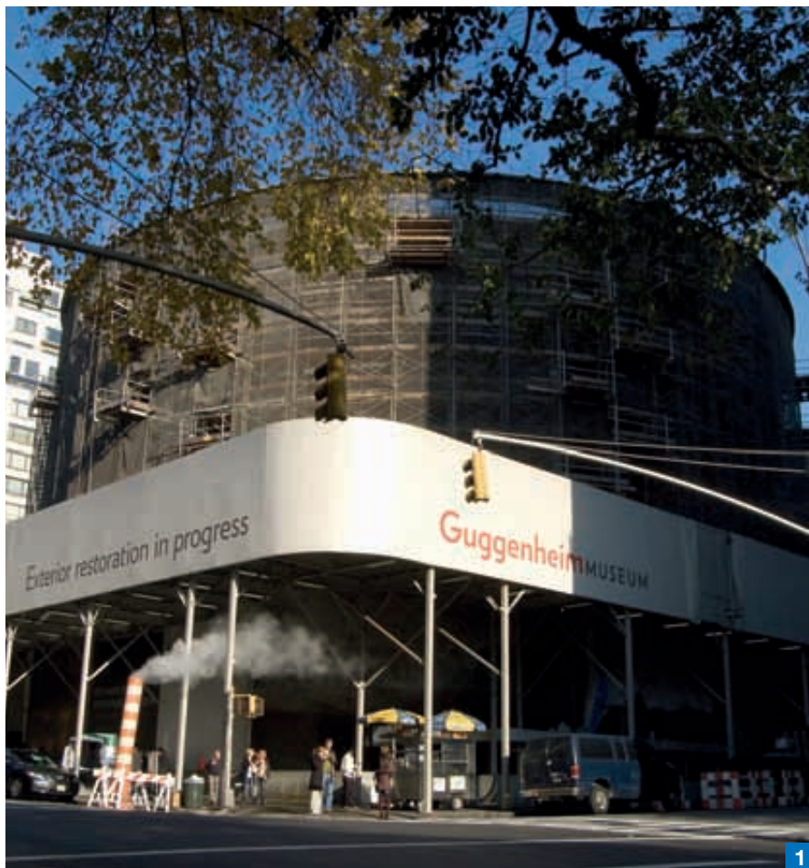
Photo 1. 2007: renovation works begins at the Guggenheim Museum.
