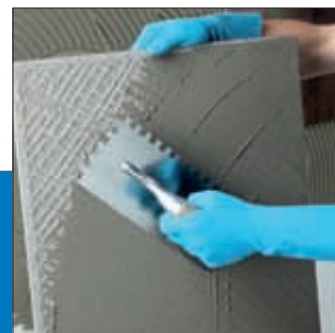
Application of the adhesive on the back of the tile
