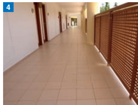
Photos 3 and 4. All the floors in the communal areas were laid with large-sized porcelain tiles using ULTRAFLEX S2 MONO.
