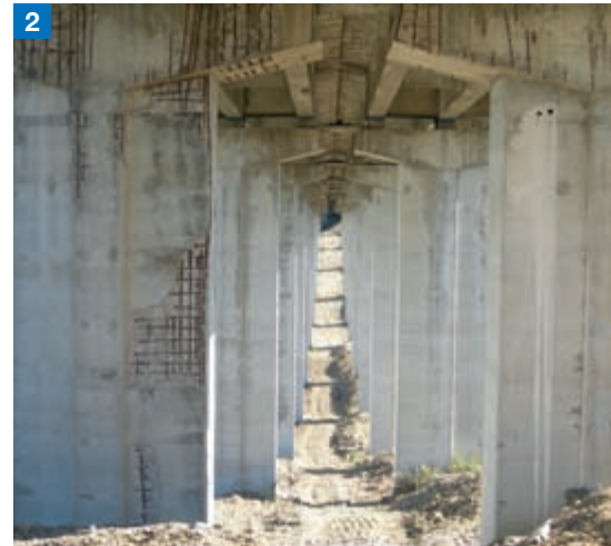
Photos 2 and 3. Beams, piles and bearing elements of the viaduct had problems of localised detached concrete, with the reinforcement rods exposed in some areas. MAPEGROUT EASY FLOW GF mortar was used to rebuild areas where the concrete had been removed.
