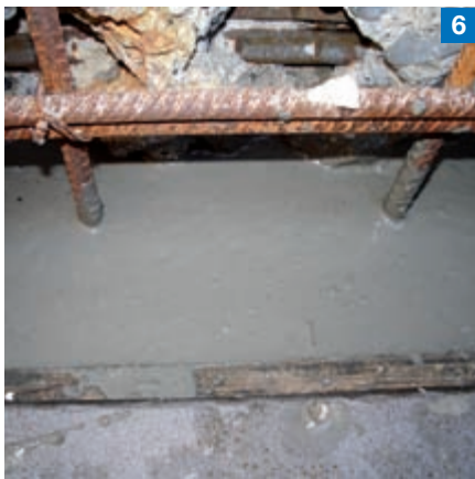
Photo 5. A steel piping was laid along the pillar and used to distribute the concrete.
