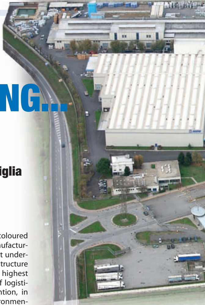
Photo 1. The start-up of manufacturing at the new plant for protective coatings for facades.
