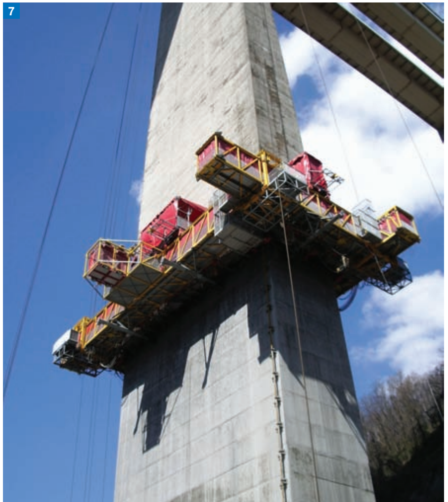
Photo 5. A steel piping was laid along the pillar and used to distribute the concrete.
