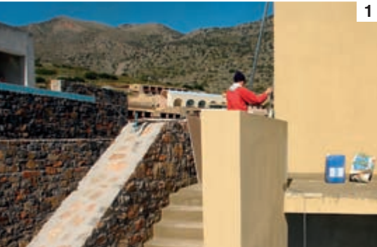
Photo 1. IDROSILEX PRONTO was applied to waterproof the external vertical surfaces.
