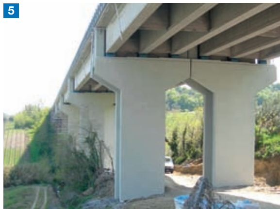
Photo 5. ELASTOCOLOR PRIMER and ELASTOCOLOR PAINT were used for the final protective coating.
