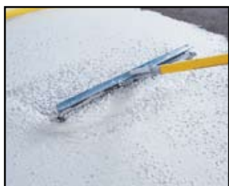
6 - Laying the product with gauge rake
