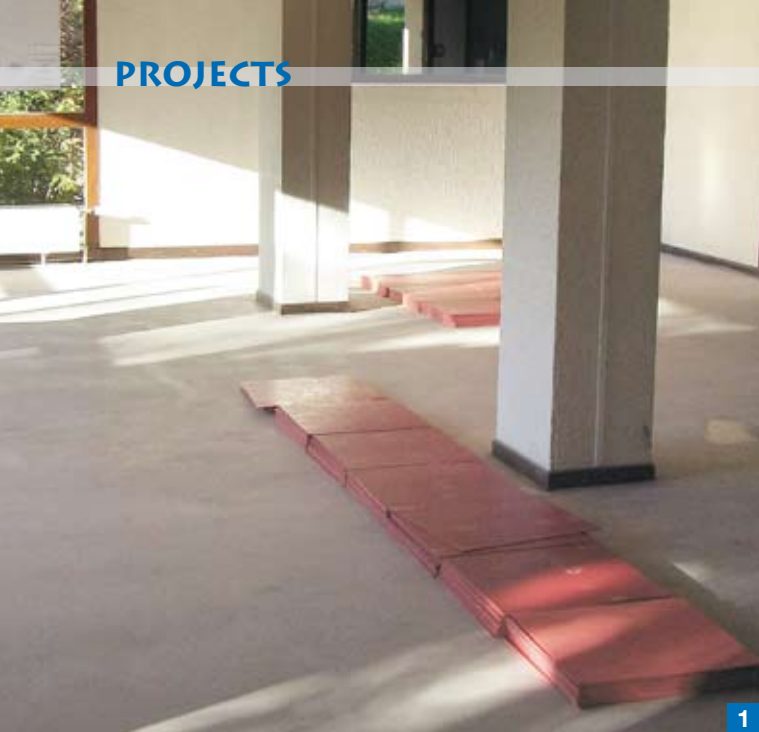
Photo 1. The floor in the refectory before laying the rubber floor covering.
