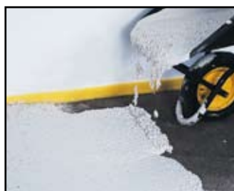
5 - Laying the product on the substrate
