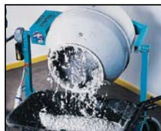
4 - Product ready for laying
