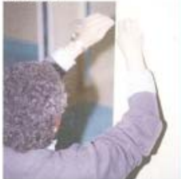
Photo 4 ADESILEX VS45 being spread on the gypsum-board
