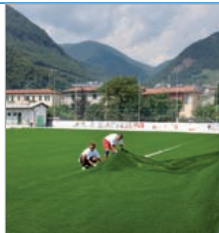
Positioning synthetic grass rolls
