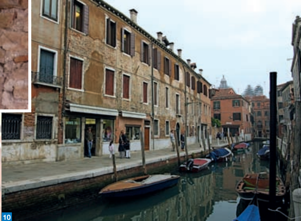
Photo 11. After completely removing the old render, a layer of MAPE-ANTIQUÉ RINZAFFO was applied. The masonry work was then evened out with MAPE-ANTIQUÉ MC de-humidifying mortar. The façade was then finished by treating it with SILEXCOLOR PRIMER and, once completely dry, 0.7 mm SILEXCOLOR TONACHINO was applied on the surface in two different colours and in white on the stringcourse.
