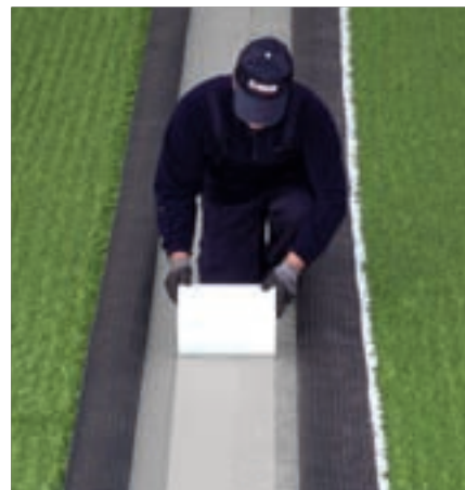
Laying the ULTRABOND TURF TAPE 100 jointing tape
