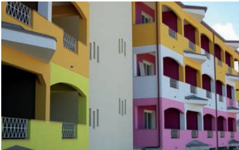
Above. A detail view of the Sikania touristic resort located in Gioiosa Marea (Province of Messina, Italy) where Mapei coatings were widely used.
