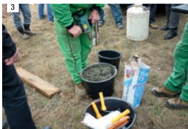
Photo 2. PLANICRETE, mixed with cement
