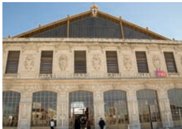
Photo 1. The new entrance hall in Saint-Charles station in Marseille.
