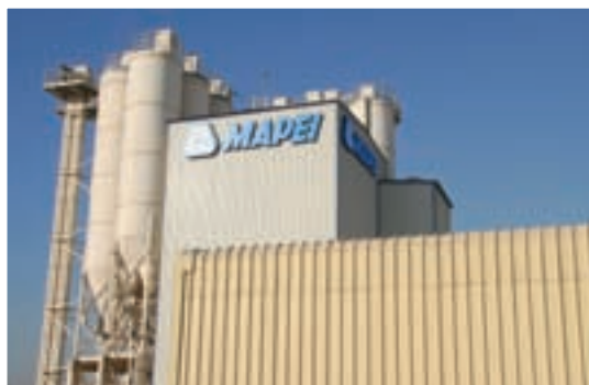
The IBS manufacturing plant in the Dubai Investments Park.
