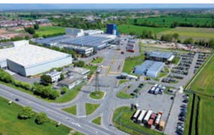
Below. A view of the Mediglia manufacturing facility and, to the side, a plan view of the route of the visit. A more detailed description of the various stops during the guided tour, which correspond to the numbers indicated in red, may be found on the following pages.
