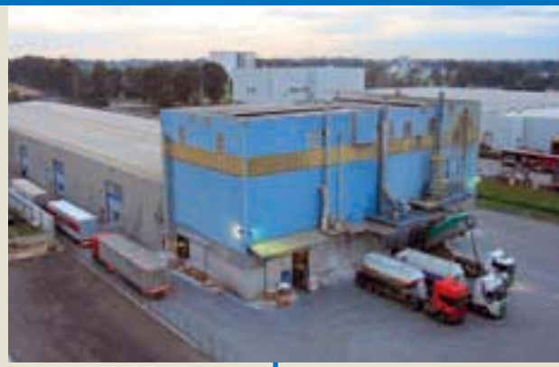
Construction of new offices and a new training area 1998 - 2002
