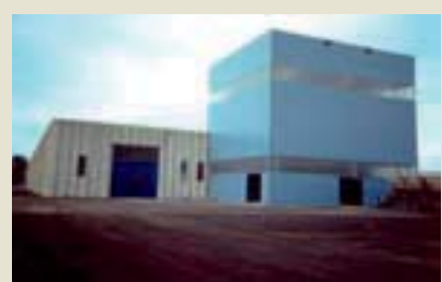
Construction of the facility and start of production with one plant 1987 - 1990
