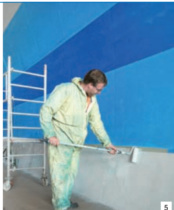
Photos 4 and 5. The final finish was applied using ELASTOCOLOR PAINT.
