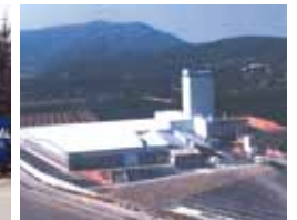
Ibermapei S.A. Amposta - Spain
