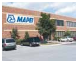
Mapei Inc. Toronto - Ontario - Canada
