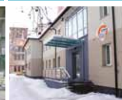
Gorka Cement Sp. z o.o. Trzebinia - Poland
