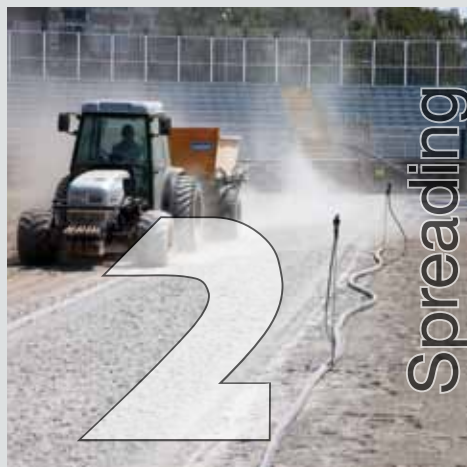
Spreading on the Mapesoil 100 with a sandblaster
