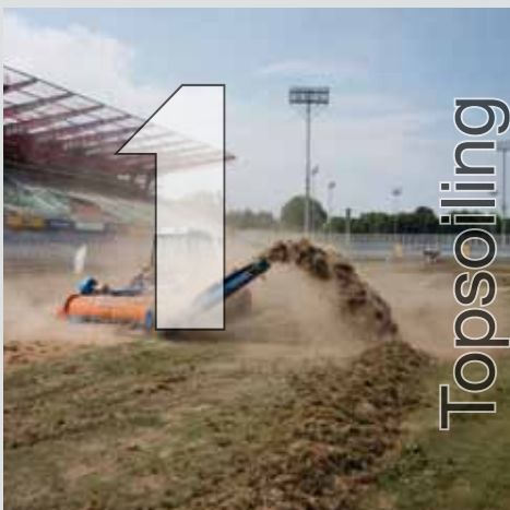
Topsoiling of the old natural grass surface
