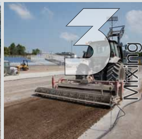
Mixing in the Mapesoil 100 with a plough
