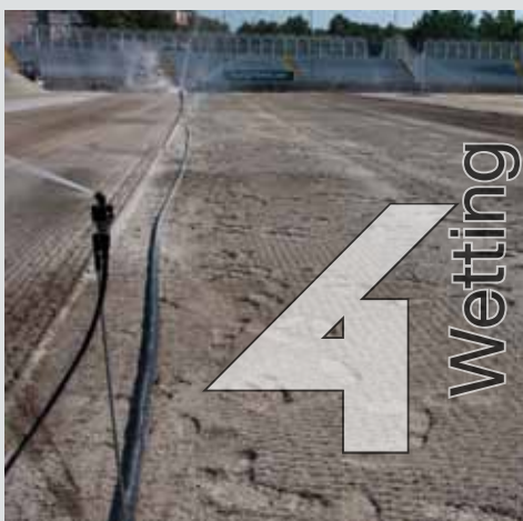
Wetting the ground
