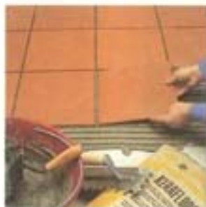
Below, more than 30.000 square metres of 7 mm thick granite tiles installed on MAPECEM screeds with KERALASTIC. The grout joints have been filled with ULTRACOLOR
