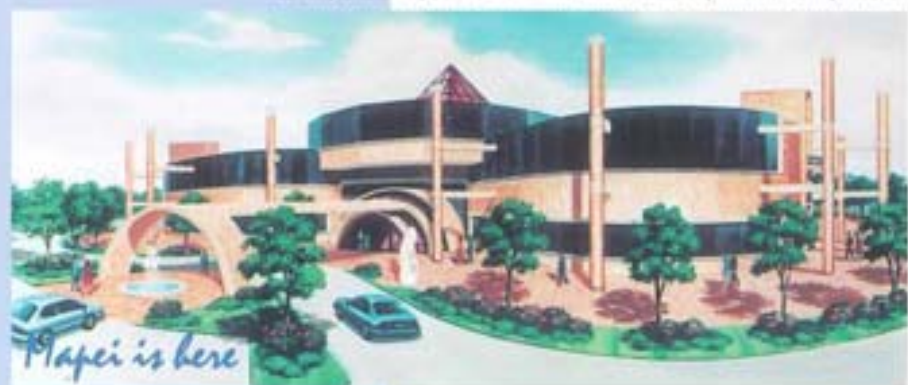
The new offices at the Garland (USA) plant during the construction phase.
