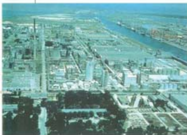
Vinavil SpA Plant - Island 12 Petrochemical - Ravenna
