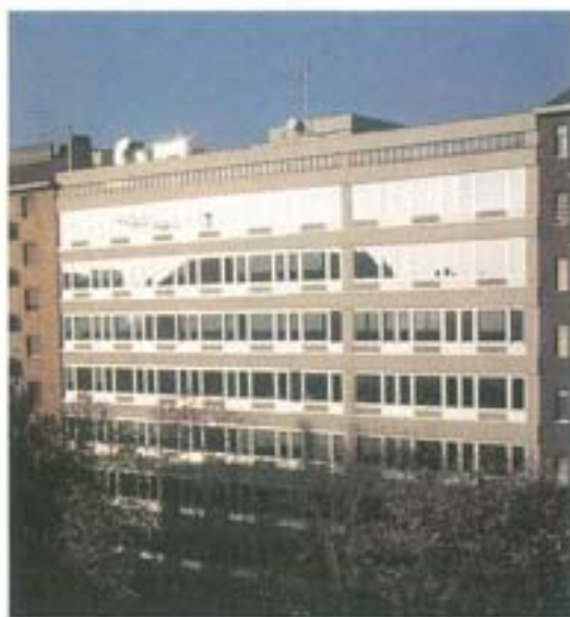
Head office of the commercial and administration offices, marketing and technical assistance - Mapei SpA Milan - Viale Jenner 4
