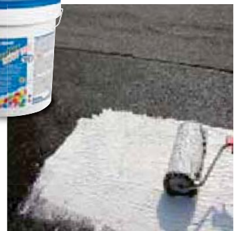
APPLYING THE MEMBRANE
