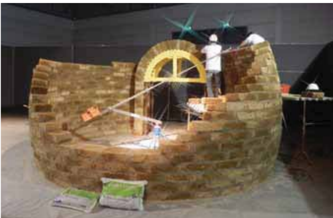
The “Carola Dome” was constructed during the trade fair by manually laying, “stone by stone”, blocks of Viterbese tuff with MALTA BASTARDA (lime-cement mortar) produced by VAGA, a subsidiary of the Mapei Group.
