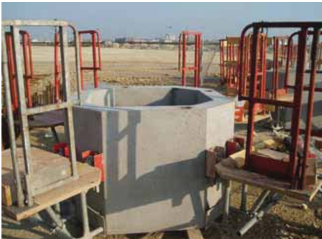
Below. Constructing and positioning the brackets on the piles at La Rochelle port on the west coast of France.
