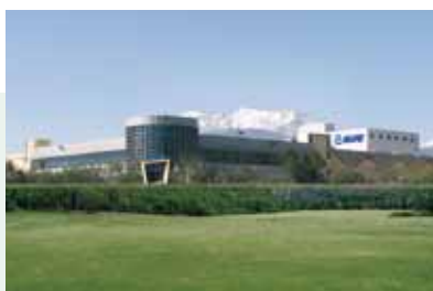
ON THE LEFT , THE MAPEI PLANT IN SAN BERNARDINO (CA) - USA, AND BELOW, FROM THE LEFT, THE GROUP'S PLANTS IN LAVAL (CANADA), GARLAND (USA) AND DEERFIELD BEACH (USA).
