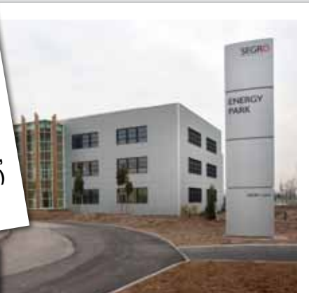
Sap Energy Park, Vimercate (MB) (LEED Gold)
