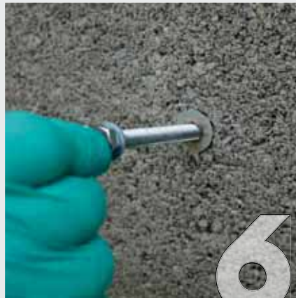
6 Rotate and insert the length of threaded bar in the hole.
