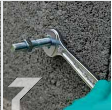
7 When the resin has hardened, the anchor is ready for use.
