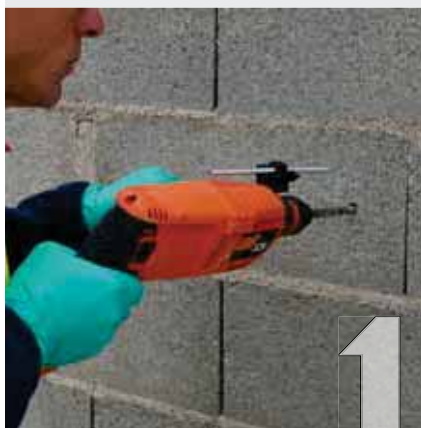
1 Drill a hole in the substrate.
