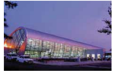
ON THE OPPOSITE PAGE AND ABOVE. Mumbai airport upon completion of work.
