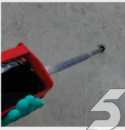
Fill the hole with resin starting at the bottom.
