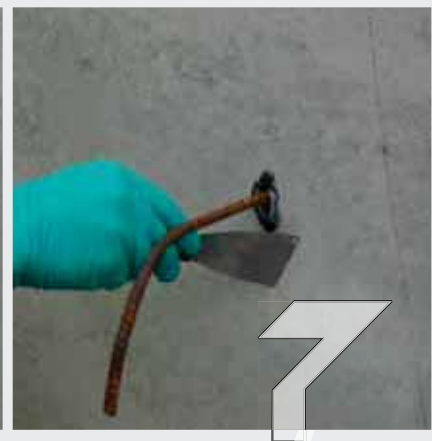
Make sure that the excess resin is expelled and remove it from around the hole.
