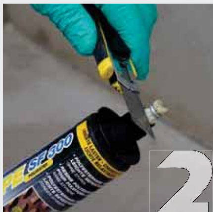
2 Before screwing the static mixer onto the end of the cartridge, cut it in correspondence with the ring.
