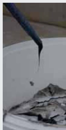
4 Pump three times and discard the resin.
