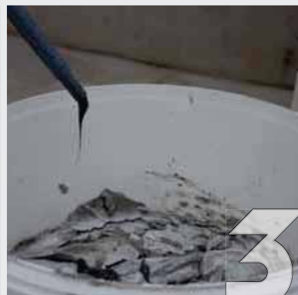
3 Pump three times and discard the resin.
