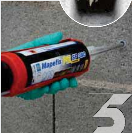
5 Fill the bush with resin starting at the bottom.
