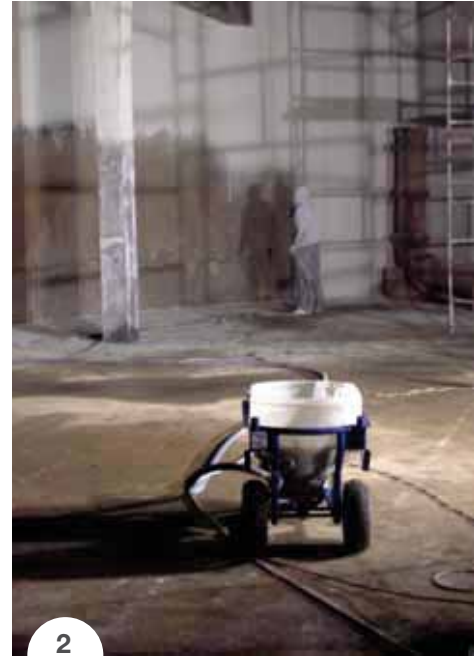
PHOTOS 1-2. MAPELASTIC was used to waterproof the internal and external concrete surfaces. Because of the size of the work, the product was applied by spray.
