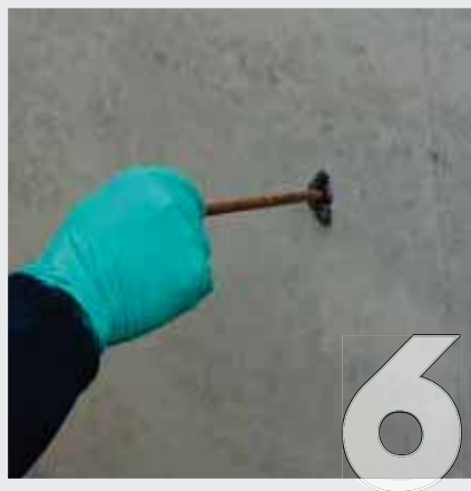
Rotate and insert the length of metal bar in the hole.
