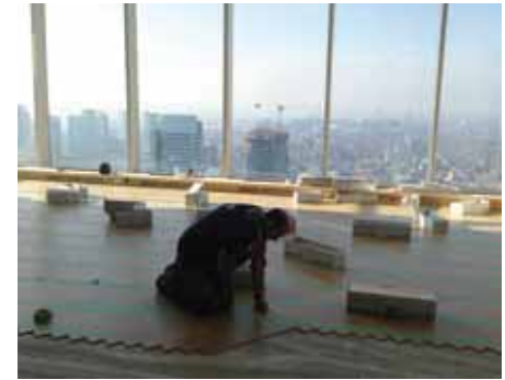
IN THESE PHOTOS. Shangri-La Hotel. The use of the one-component adhesive ULTRABOND ECO 995 allowed for perfect laying of the wooden floors while also acting as a soundproofing layer.
