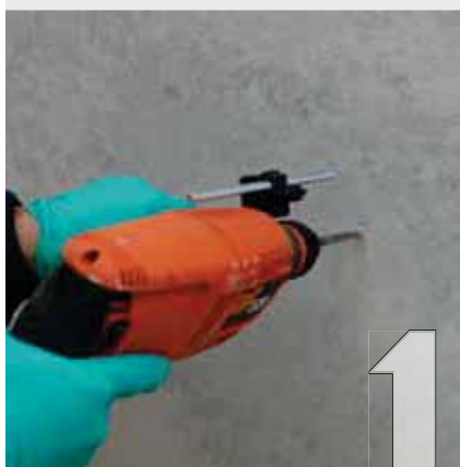
1 Drill a hole in the substrate.
