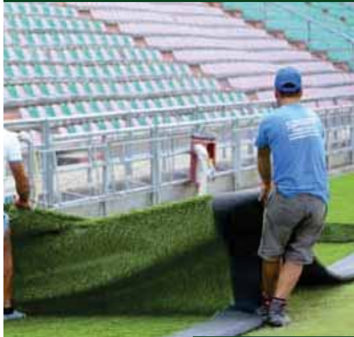
Laying of synthetic grass around the edge of the pitch.
