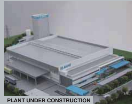
PLANT UNDER CONSTRUCTION
