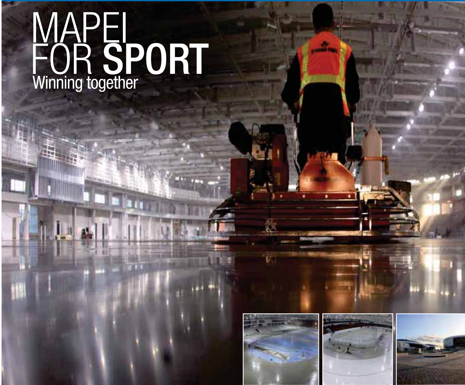
Minsk Ice Palace, Belarus Building concrete floorings with Mapecrete System
