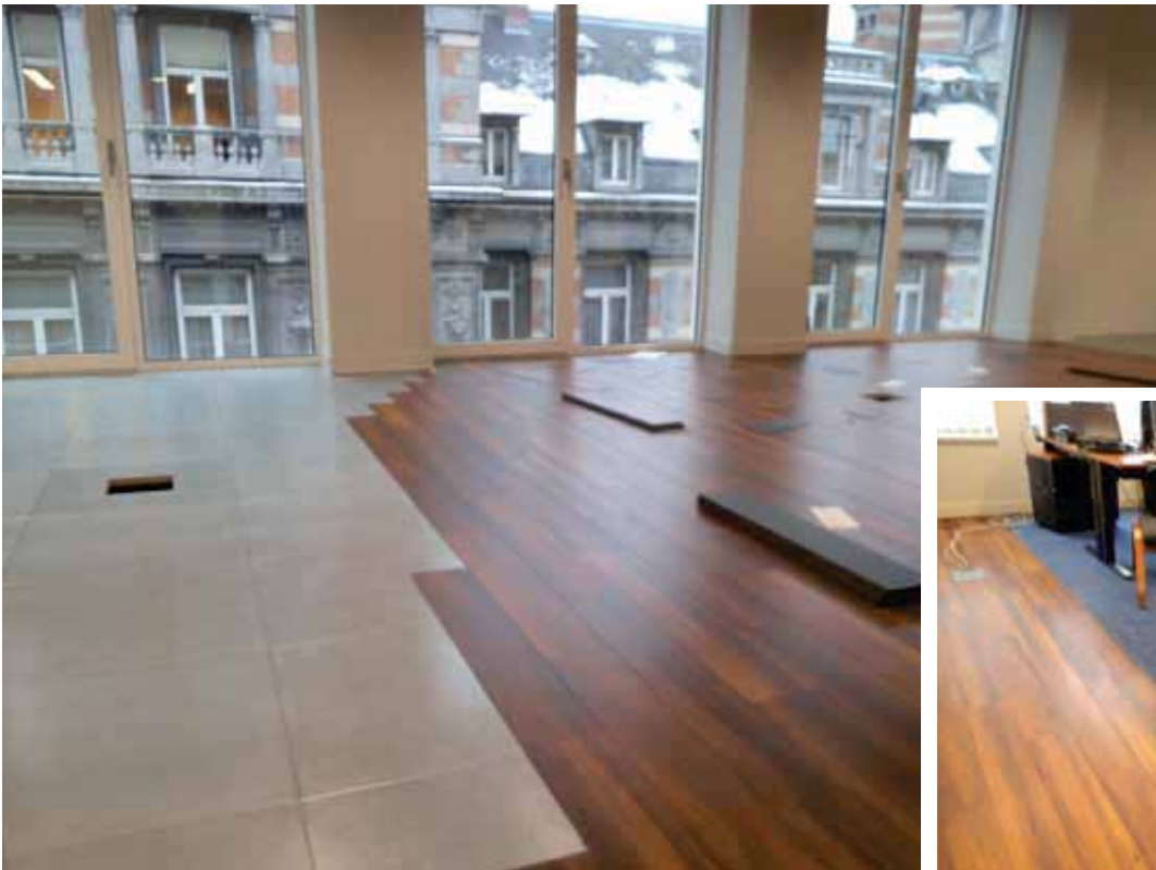
LEFT. Before installing the flooring, ULTRABOND ECO TACK LVT must turn from white to transparent. BELOW, RIGHT. The floor once installation had been completed.
