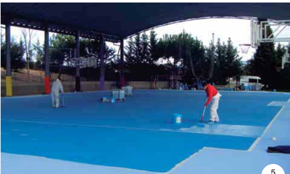
PHOTOS 3 and 4. Applying MAPECOAT I 600 W before laying MAPECOAT TNS BASE COAT.
