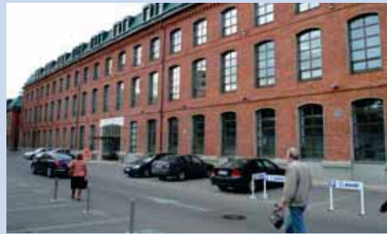
LEFT. ZAO Mapei has its headquarters and offices in downtown Moscow .
