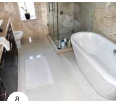
PHOTOS 6, 7 and 8. The materials for substrate preparation were mixed on the penthouse patio. The TOPCEM PREMIX mud bed was allowed to cure for two days, and then ULTRATOP WHITE was laid on the floor substrates in the kitchen, dining-room, corridors and bathrooms.
