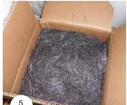
PHOTO 2. The cementitious flooring made with ULTRATOP WHITE added elegance to the penthouse apartment at 198 Aquarius Mews in Vancouver. PHOTOS 3, 4 and 5. The floor screed was built using TOPCEM PREMIX, PLANICRETE and stainless steel fibers. It was laid over a radiant heating system.
