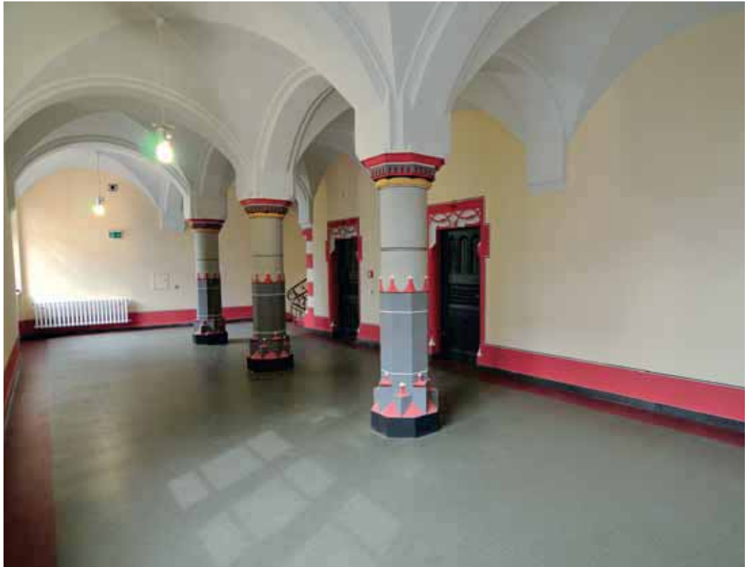
LEFT. Most of the floorings in the renovated areas were covered with linoleum bonded with ULTRABOND ECO 520.
