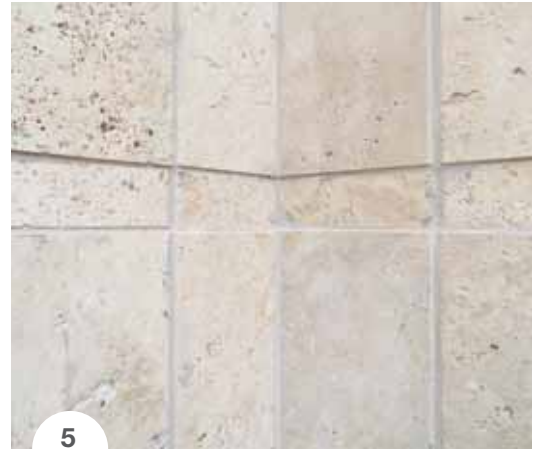
PHOTO 4. Travertine slabs were also installed on the outside columns with GRANIRAPID.
