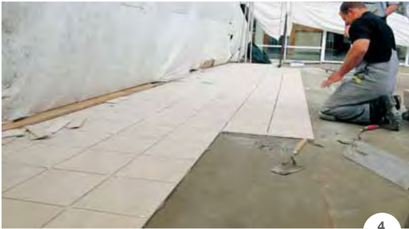
PHOTO 4. The porcelain tile floorings were bonded with KERAFLEX MAXI S1 adhesive.
