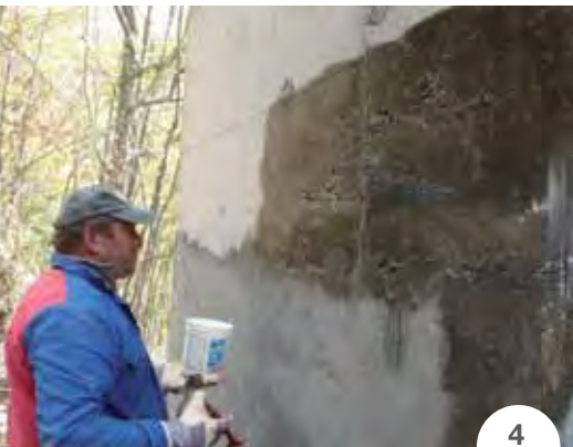
PHOTO 4. The concrete surfaces were treated with MAPEWRAP PRIMER 1 and levelled with MAPEWRAP 12 epoxy grout.
